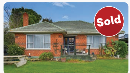
212 Walnut Avenue, Ashburton
