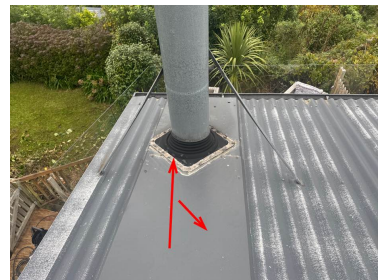
Chimney penetration flashing
