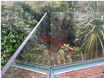
Glass Bella strain leaning out
