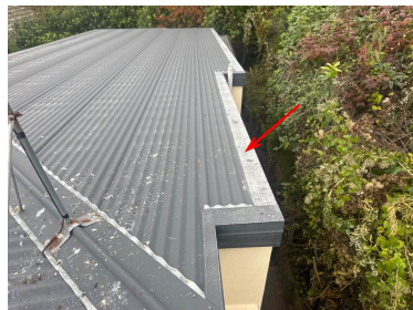
Barge flashings
