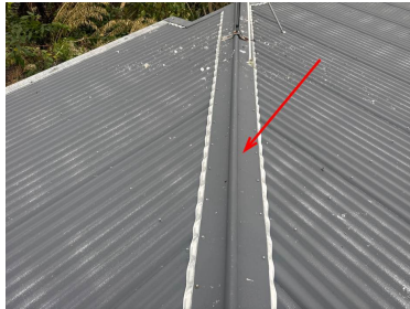
Ridge and hip flashings
