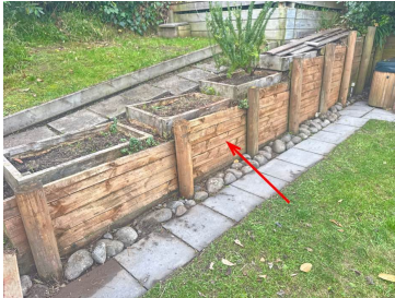
Glass Bella strain leaning out
