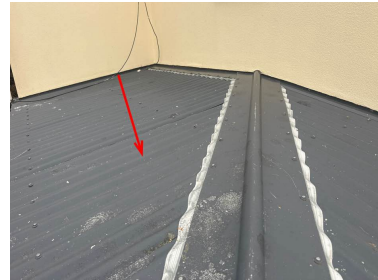
Corrugated colour steel roofing
