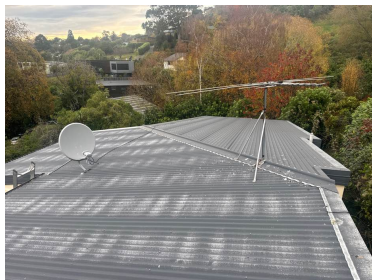
Ridge and hip flashings
