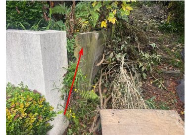
Retaining wall leaning out
