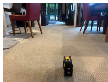
Kitchen dining living room floor level within 20 mm
