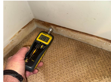
Significant water damage backing onto the shower
