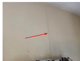
Crack above doors opening to deck end of house
