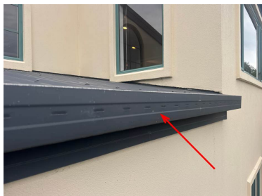
Colour steel gutter system
