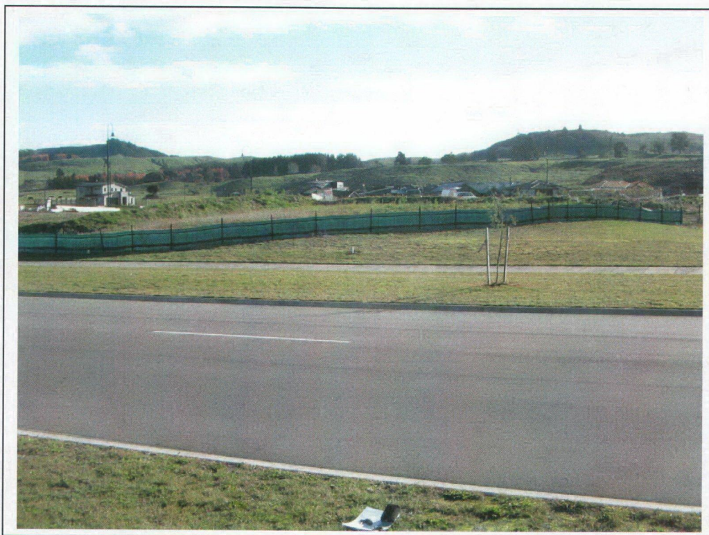
Photo 4 – View of Lot 31 where the proposed rock retaining wall (the shade cloth bisects Lot 31)
