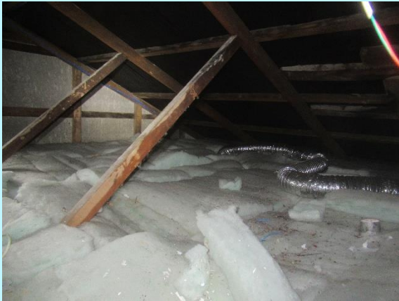
Traditional timber framing with several old remedial repairs provides the roof support
