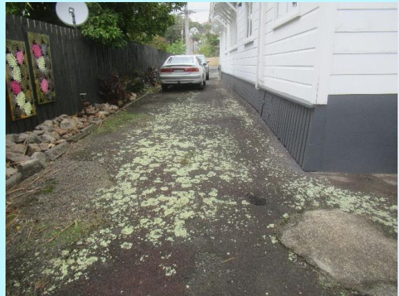
Timber base boards with gaps allow good crossflow ventilation in the timber subfloor
