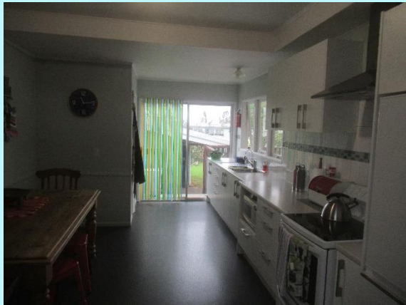
Kitchen with mechanical ventilation installed over the stove
