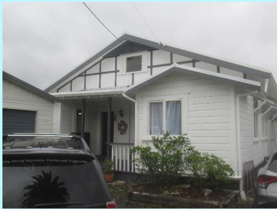
The main entry is located at the front south facing elevation
