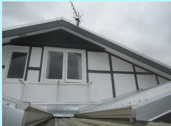
Windows provide passive ventilation and natural light into the attic conversion
