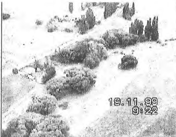
Site of access road crossing Lots 1 & 2
