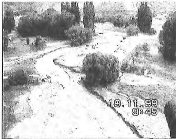
Swann Rd and adjacent washout
