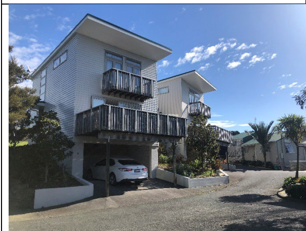
RECENTLY COMPLETED UNITS SHOWING GARAGING
