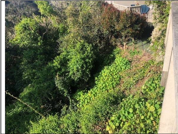
COMMON AREA TO THE NORTH OF PU-18 REQUIRES EXTENSIVE MAKING GOOD.
