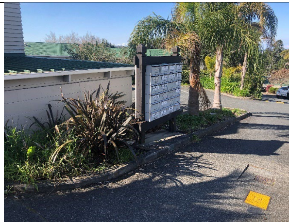
LETTER BOXES IN GOOD ORDER ANOTHER SLUICE VALVE SURROUND TO BE REPLACED LANDSCAPING REQUIRED
