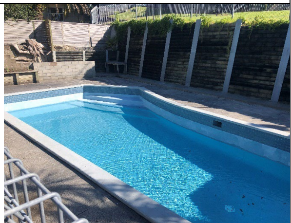
RECENTLY PLASTERED POOL SURFACE RECENT RETAINING WALL
