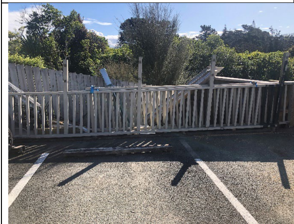
DEMOLITION DEBIS TO BE REMOVED PU-19, AU-43
