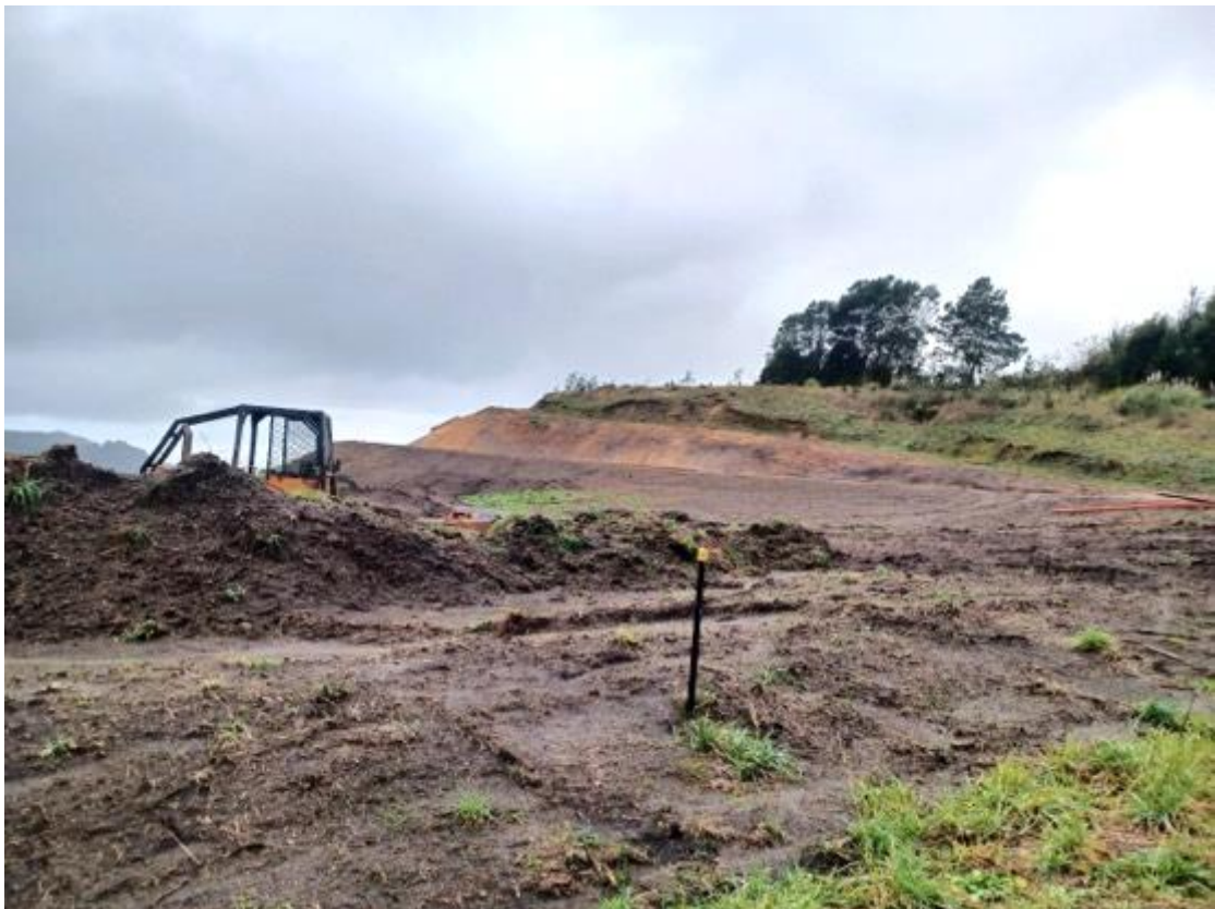
Figure 6: View on the proposed building platform and eastern slope
