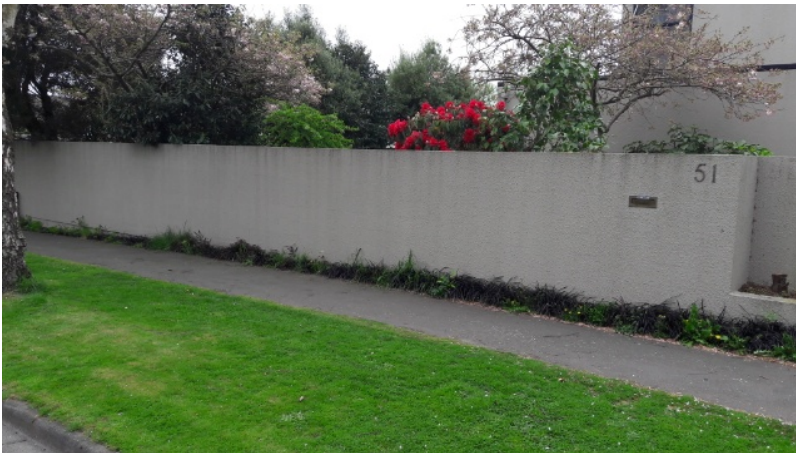
Figure 2 : Plaster block fence- No visible EQ damage - No action required.
