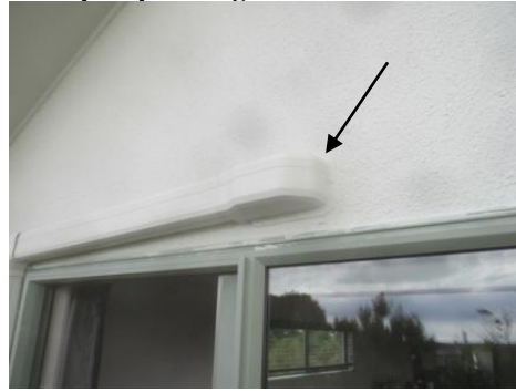
Heat pump through lintel
