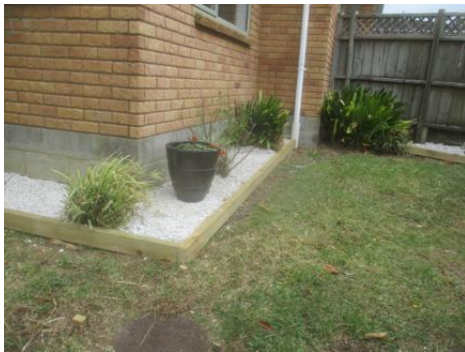
Cladding in contact with grounds
