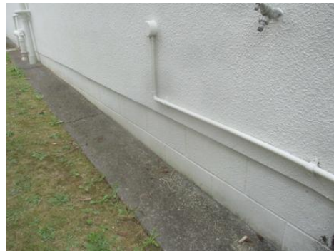
Cladding in contact with grounds
