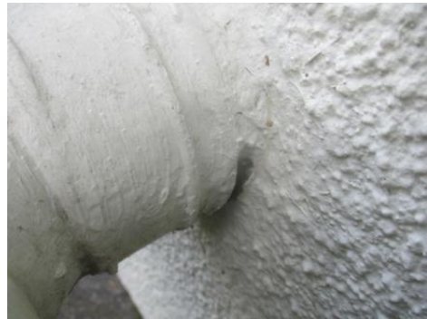
Keep penetrations well sealed
