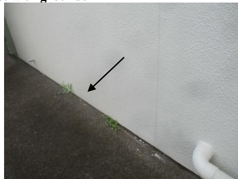
Cladding in contact with grounds
