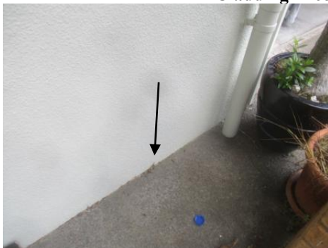
Cladding in contact with grounds
