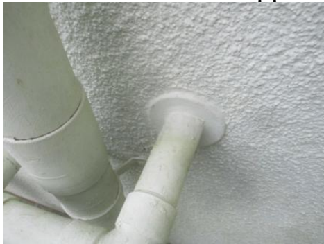
Keep penetrations well sealed
