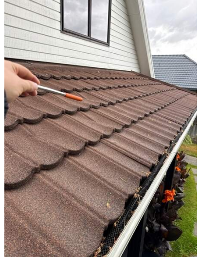
#98: Tile dents - Southern elevation
