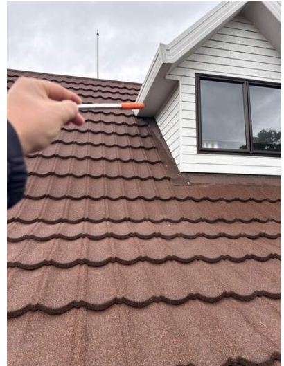
#106: Cracked eave lining - Western elevation
