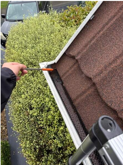
#103: Surface rust - Western elevation
