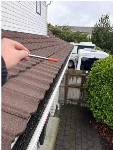
#100: Popped nails - Eastern elevation
