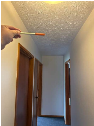
#136: Smoke alarm required - Hallway
