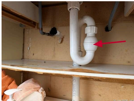
#47: Leaking waste.
