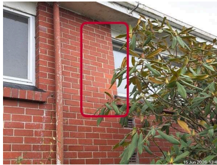
#86: Repairs visible eastern face.
