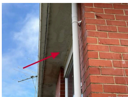
#131: Mould staining.
