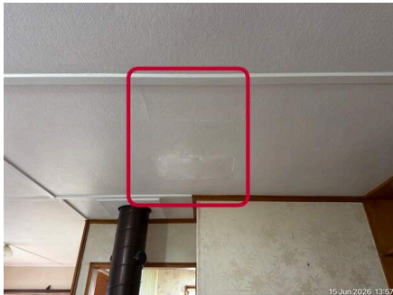
#16: Patching in the living room.
