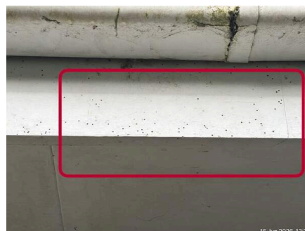
#129: Borer holes in the Fascia.
