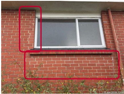
#85: Brick repairs visible to the eastern face.
