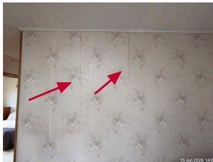
#22: Multiple cracks.
