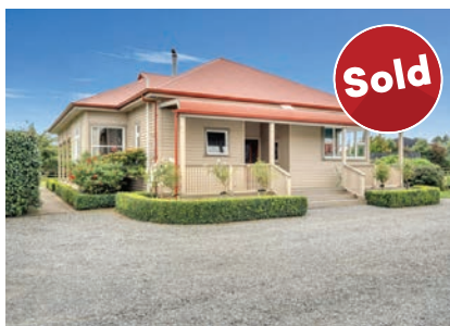
72 Rakaia Barrhill Methven Road, Rakaia
