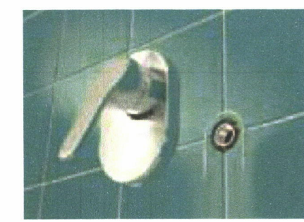
Run a bead of silicone sealant around the mixer unit on the tiles extending below the bottom of the pipe aperture.
