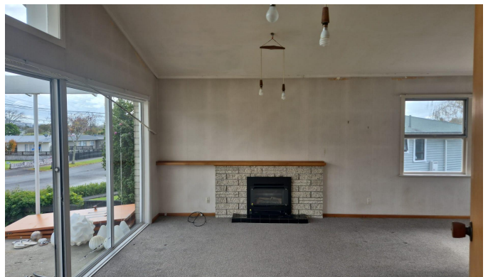
Stage 4 - Sheeting fully removed
