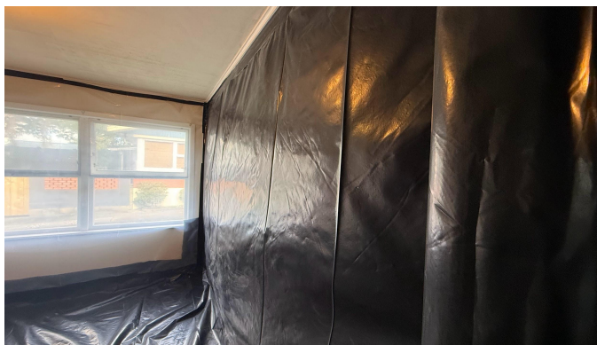
Stage 2 - Sheeted walls visually clear
