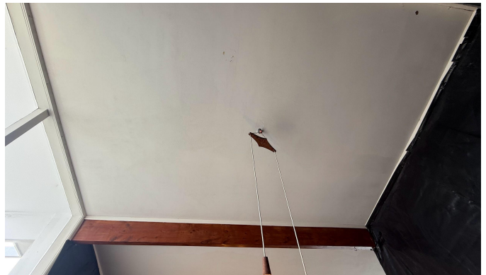
Stage 2 - Textured coating removed from living room ceiling
