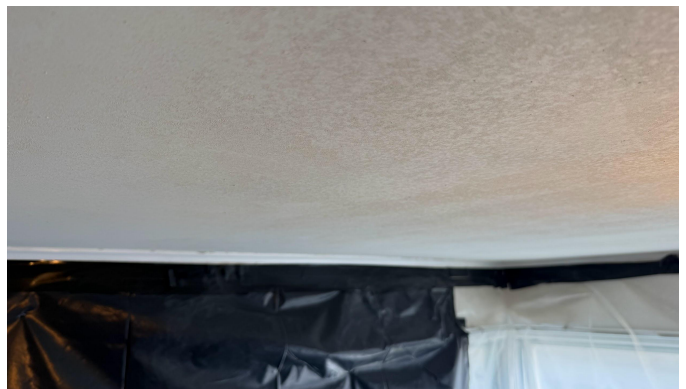
Stage 2 - Plasterboard in situ visually clear.
