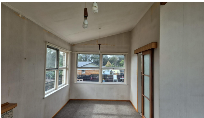
Stage 4 - Sheeting fully removed
