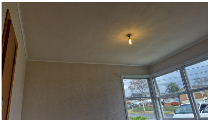
Stage 4 - Ceilings encapsulated.
