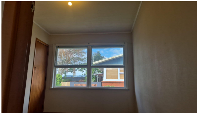
Stage 4 - Sheeting fully removed
