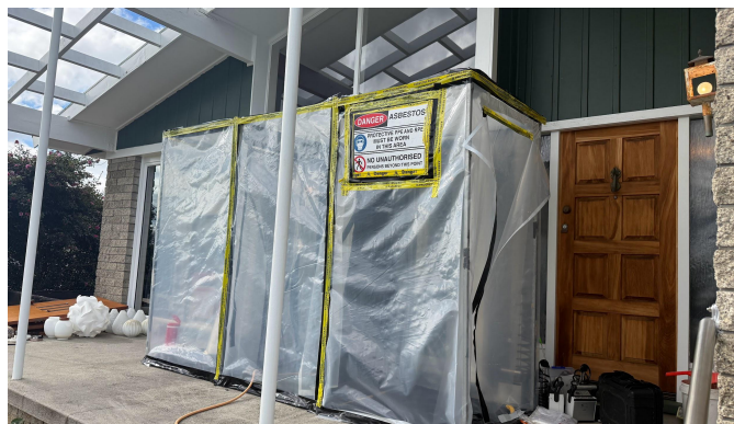
Stage 1 - Decontamination Unit/Area
