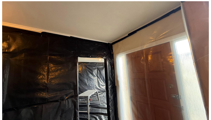
Stage 2 - Overview of enclosure - Hallway
