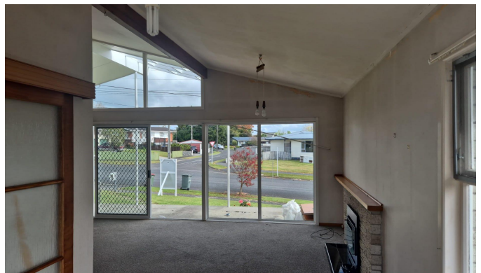
Stage 4 - Sheeting fully removed
