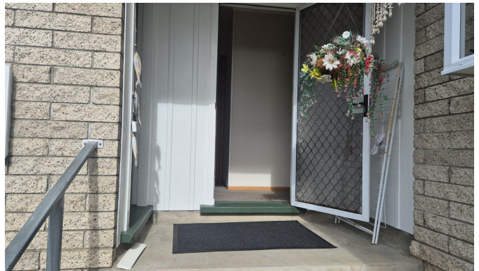
Stage 4 - NPU 1 fully removed.
