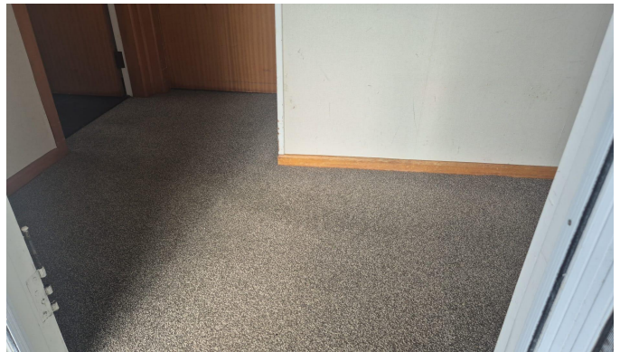
Stage 4 - Sheeting removed from floors.
