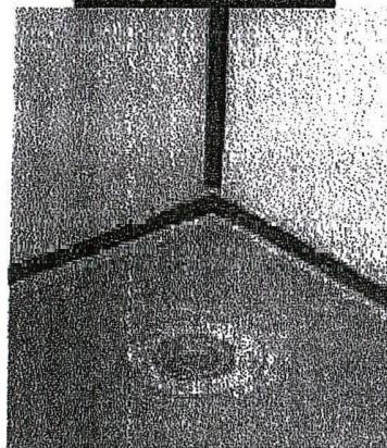
Bathroom wall waterproofed with Mapegum WPS and Mapeband
