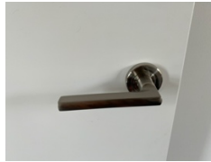
Internal Door Hardware
