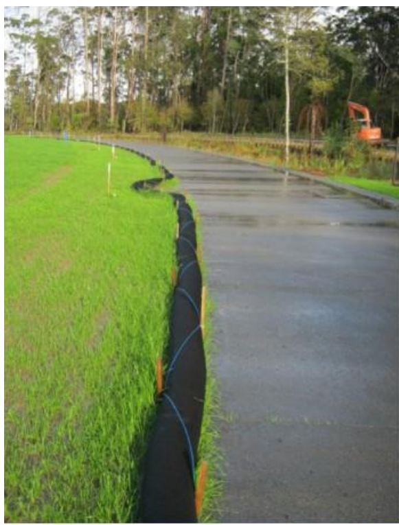
Silt sock used to provide control during final landscaping works (Source: Erosion Control Ltd)
