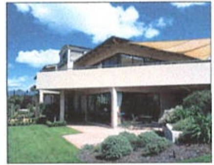
This Nelson home is finished with Rockcote Architectural Coatings' LiteRock Solid Plaster System. A pre-coloured polymer render and Finecoat give a crack-resistant, soft-patina effect to this home, designed by Christchurch architect John Davey.
