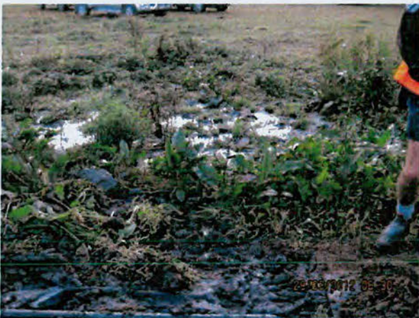
Photo 1 showing surface ponding on the north-east side of the mound.
