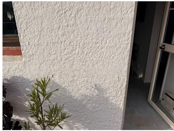
Photo 4. View of repaired cladding.
