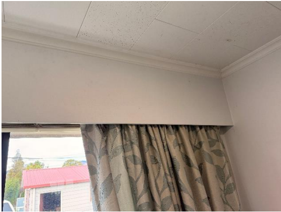
Photo 7. Internal lining has been repaired.
