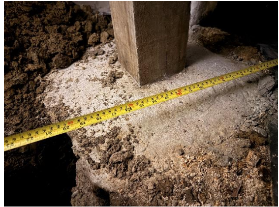
Photo 8. Internal pile footing size.
