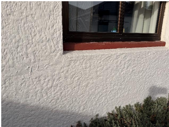
Photo 3. View of repaired cladding.
