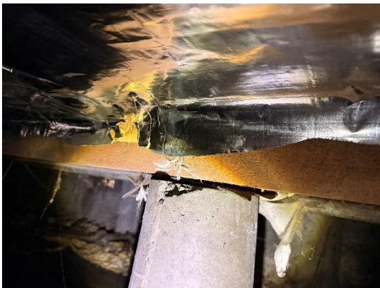
Photo 11. View of internal pile.
