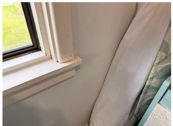
Photo 6. Internal lining has been repaired
