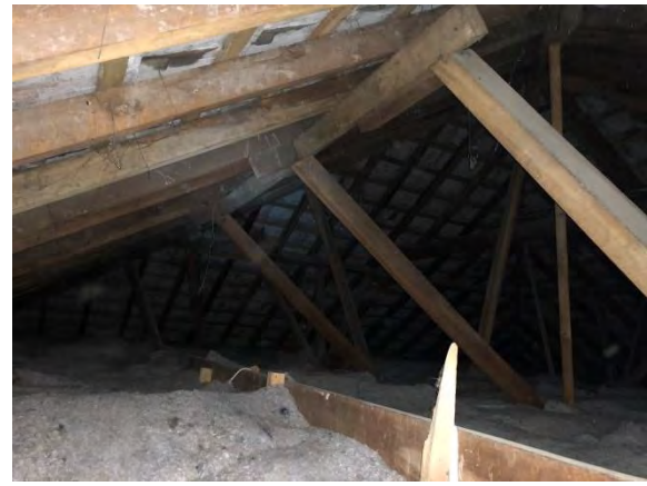
Photo 11. View of the roof cavity.
