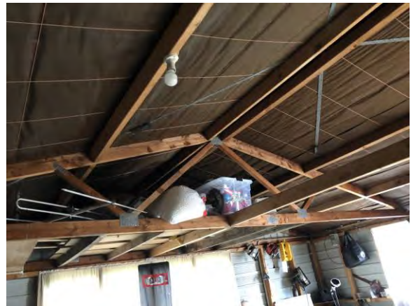
Photo 17. View of the garage roof structure.
