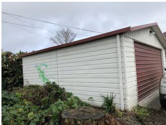
Photo 14. Southeast view of the garage.
