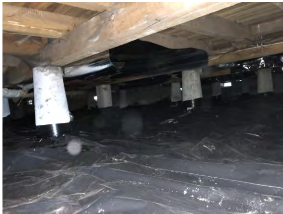
Photo 12. View of the subfloor.
