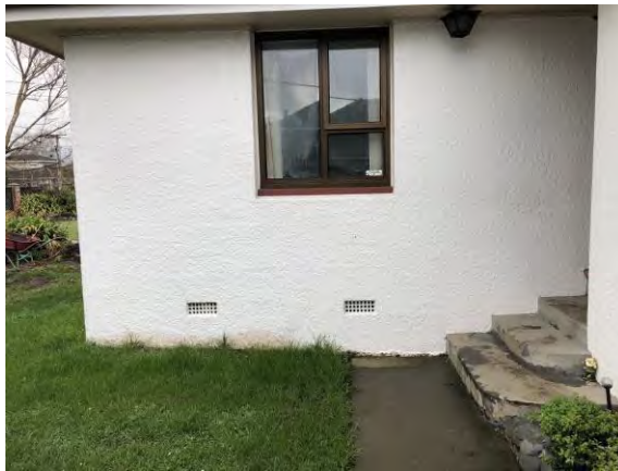
Photo 4. Perimeter concrete foundation covered by stucco plaster.
