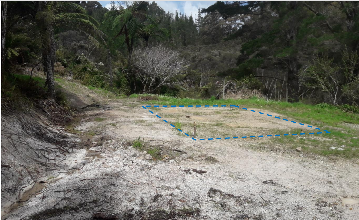
Looking south (approx.) across proposed building platform. Bank below building platform to top right of image (grassed area). Non-certified fill material encountered at far corner of build platform.
