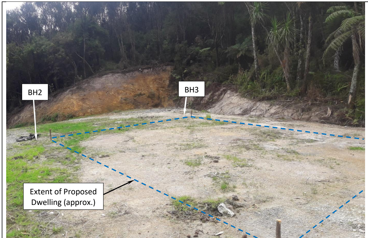
Looking northeast (approx.) across proposed building platform. Pegs denote approximate dwelling location. Note the steep cut bank with exposed soils and open drain at base of slope, top of image.
