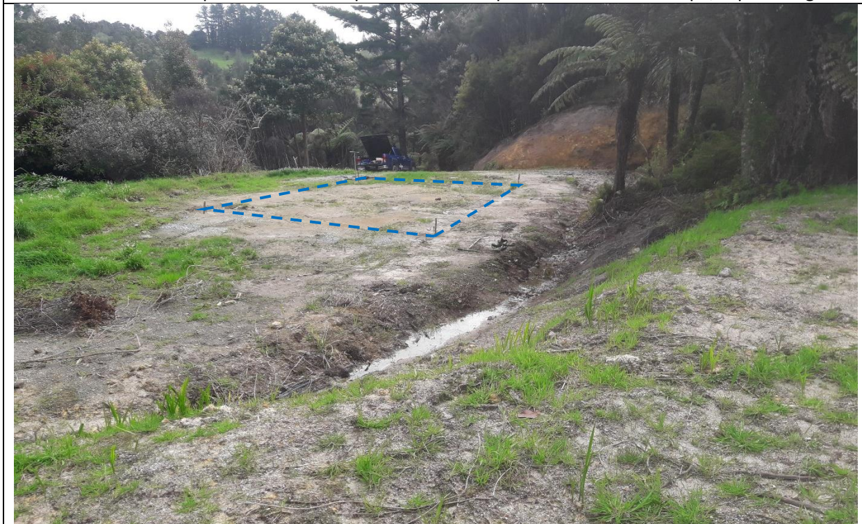
Looking north (approx.) across proposed building platform (dashed line). Note open drain at base of slope that extends around the perimeter of the propose building platform.
