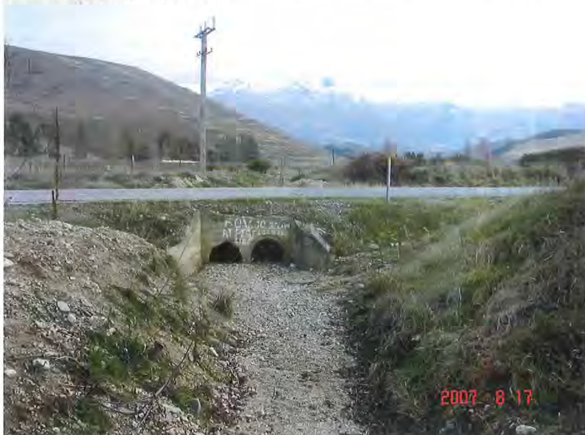
Figure 5: State Highway 6 culverts from downstream
