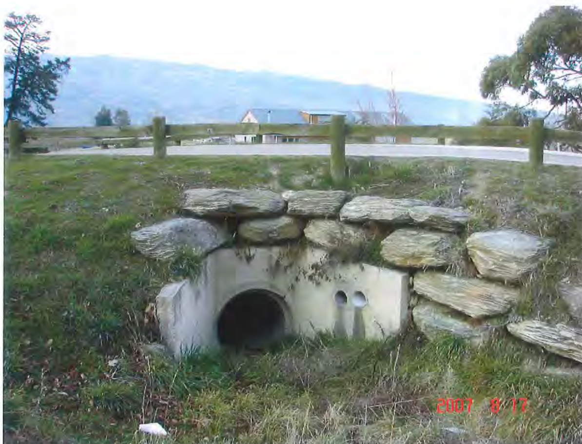
Figure 6: Entrance to Pisa Moorings Road 900mm diameter culvert. Note road higher over culvert than left and right
