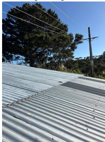
Some corrosion to sheet.
