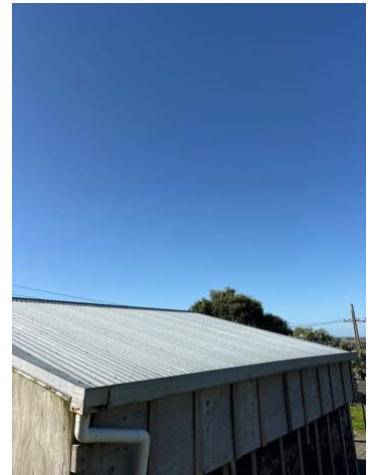
Roof good to this area.
