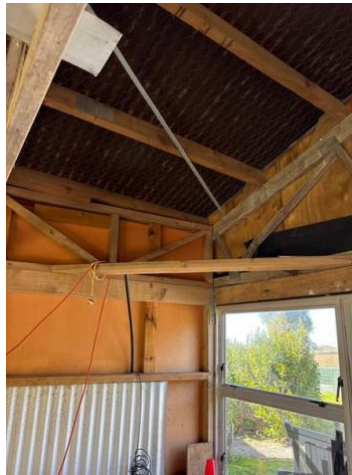
Adequate bracing for age.
