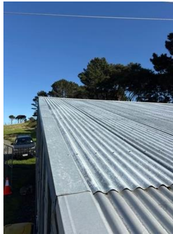
Roof overall good for age.
