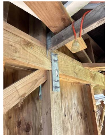
Adequate bracing to structure.
