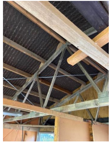
Trusses in good condition.
