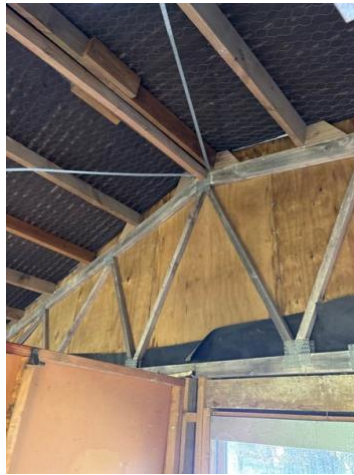
Roof bracing visible.
