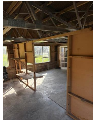
Load bearing walls overall good.
