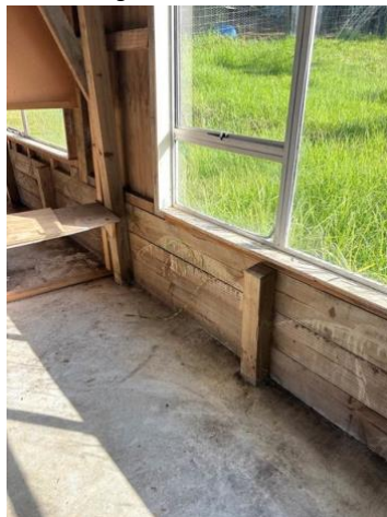
Retaining overall good.
