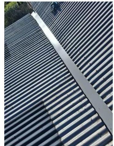
New gutter in good condition.
