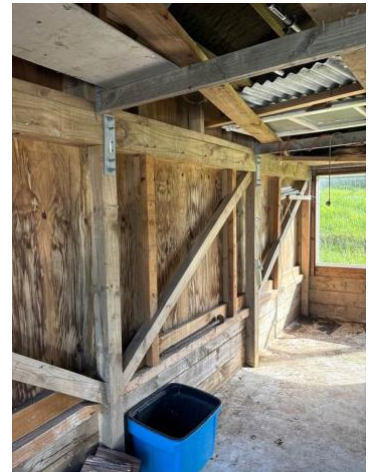
Adequate bracing to structure.
