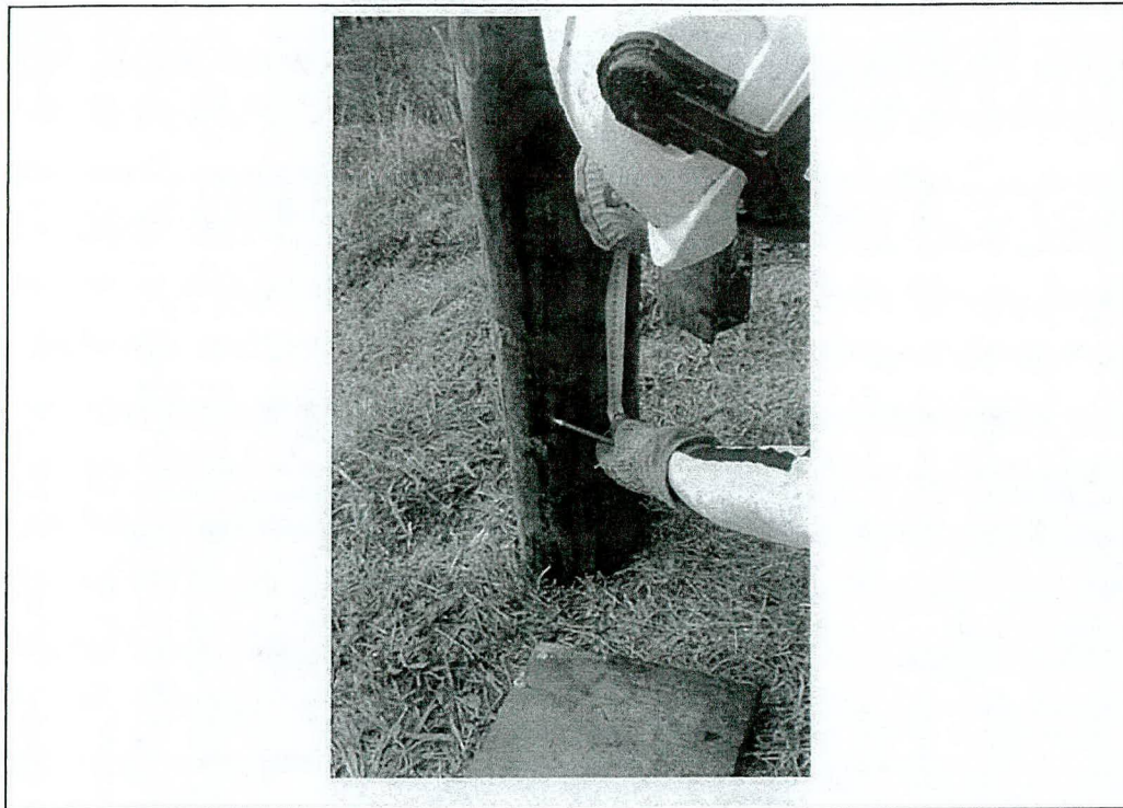
Photo 3 – Checking the set mm per blow
