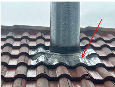
Chimney penetration flashing
