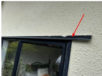
Window head flashing
