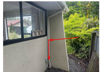
All downpipes discharging into stormwater as intended
