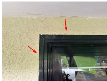
All windows well as sealed around the edges
