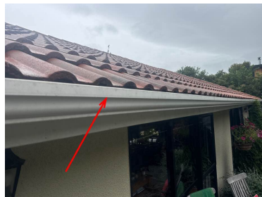
Plastic gutter system
