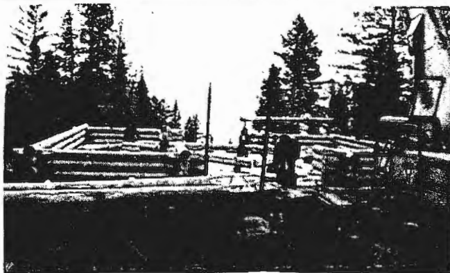
Site of the Del Radomske built 1800 sq foot house at Kelowna, overlooking Okanagan Lake.
