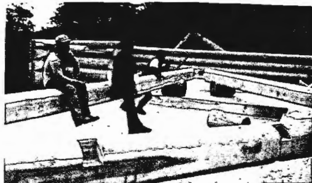
Assembling roof trusses for the 1800 sq foot Del Radomske built home.
