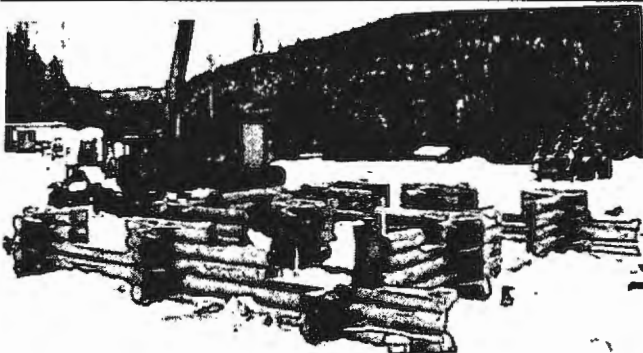
And the snow lay all about ... the Del Radomske building site - the first that brought Bruce Jamieson flying back to NZ for a few weeks in January. A 1000 sq ft house is shown being packed into a container for shipping to Japan.
