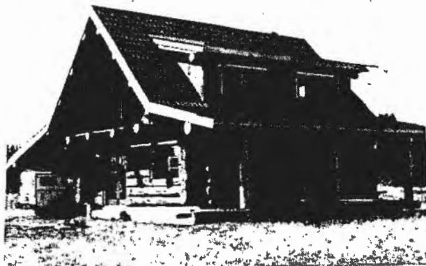
The McMillan log home at Ohakune. The log work was done by the 1983 Course at the Ohakune School of Log Building tutored by Del Radomske. The log work has been treated with Sik's Oil, or Cetol, a product imported from one of the Scandinavian countries.
