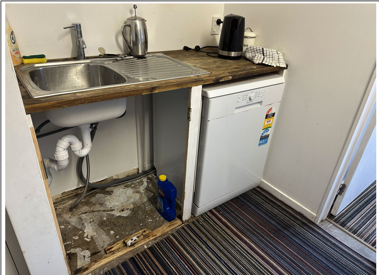
6.21 Overview of Kitchenette backing onto bathroom in Unit 28
