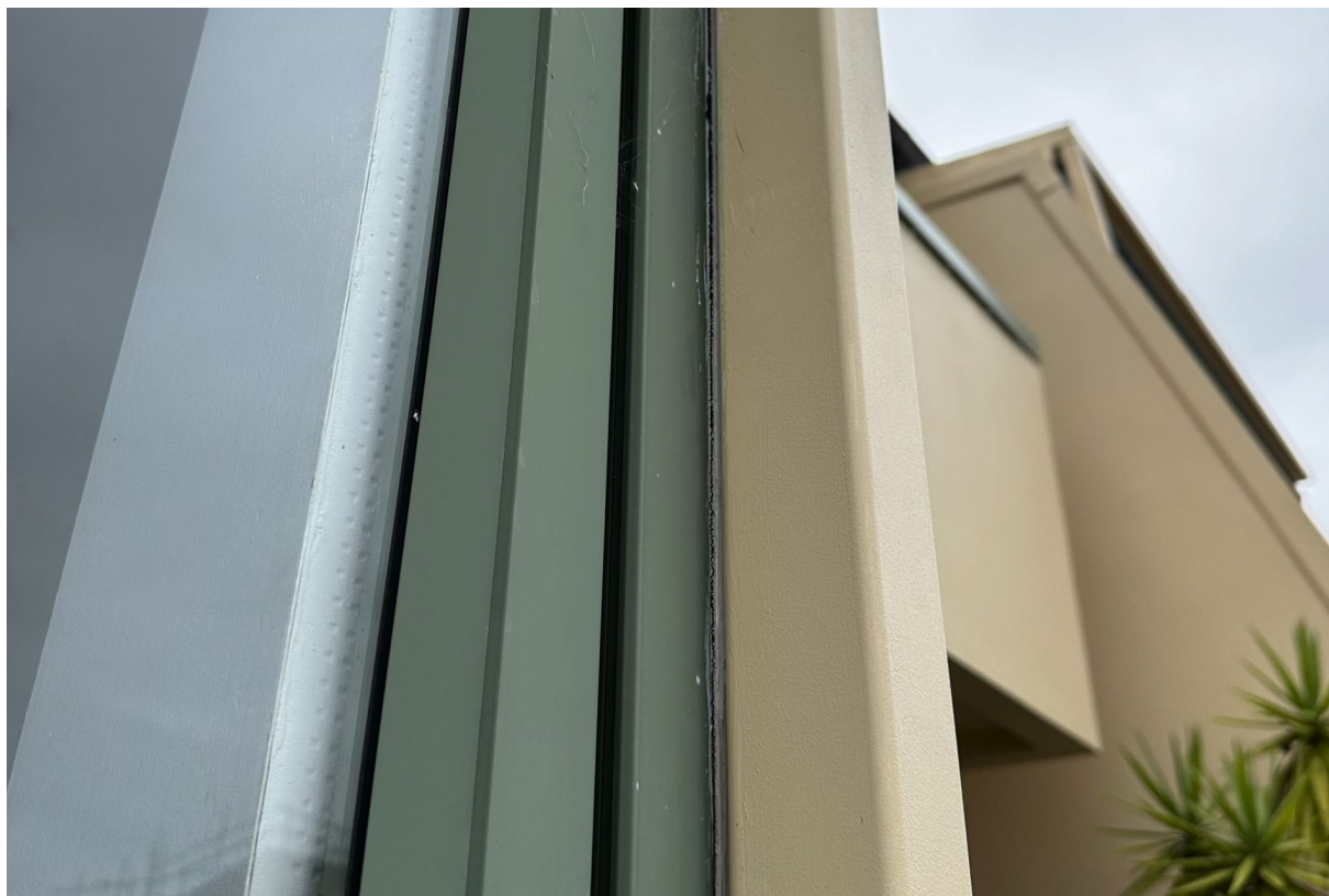
6.2 Open flashing junction beside window joinery
