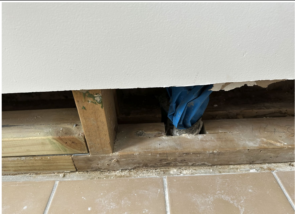
6.8 Change in framing along intertenancy wall between Unit 27 and Unit 28
