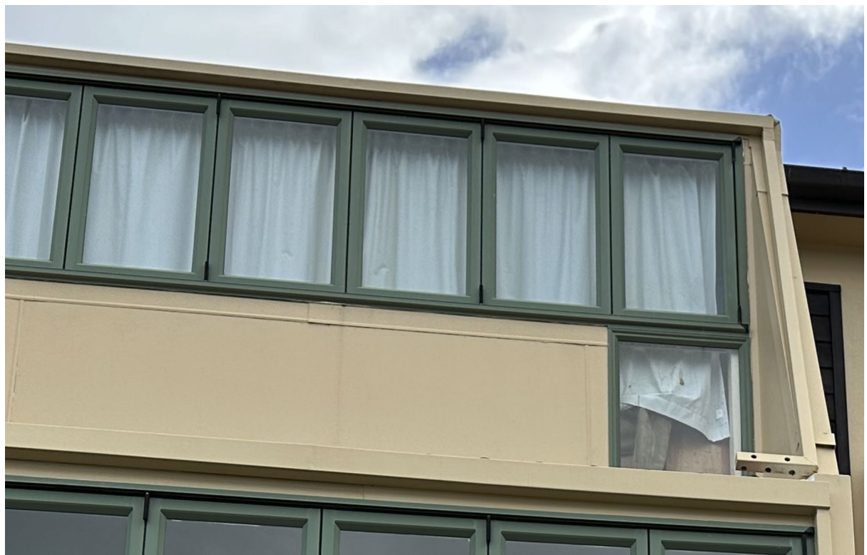
6.13 Overview of Level 2 Bedroom window joinery in Unit 28
