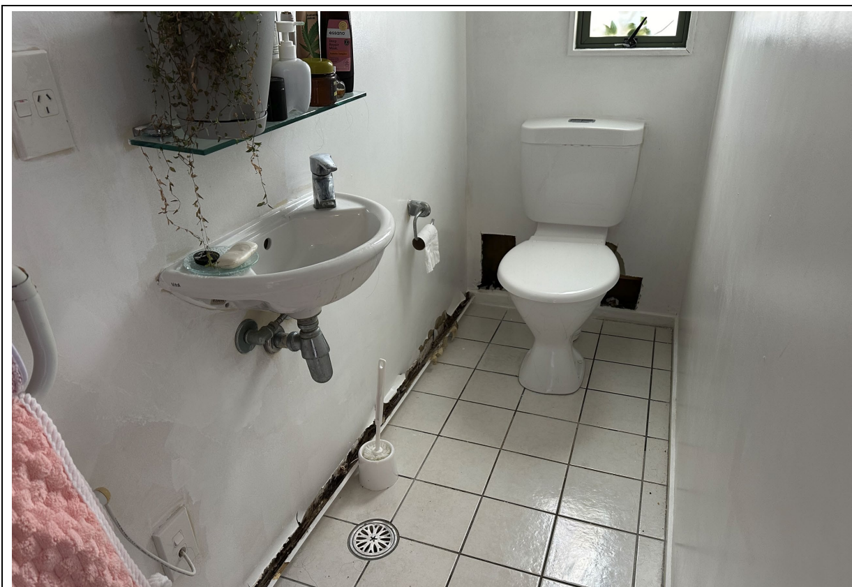
6.17 Overview of Ground Floor Bathroom in Unit 28 facing towards external wall
