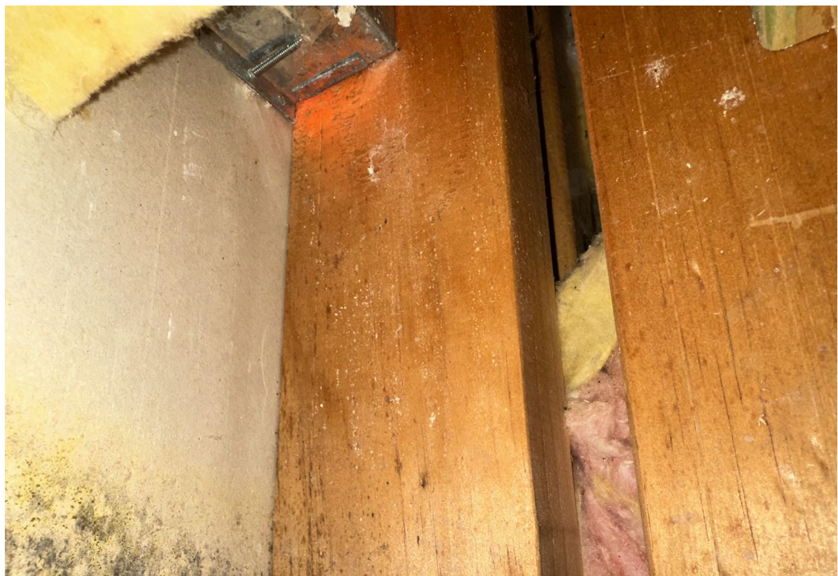
6.12 No visible water staining from above evident within the intertenancy wall cavity
