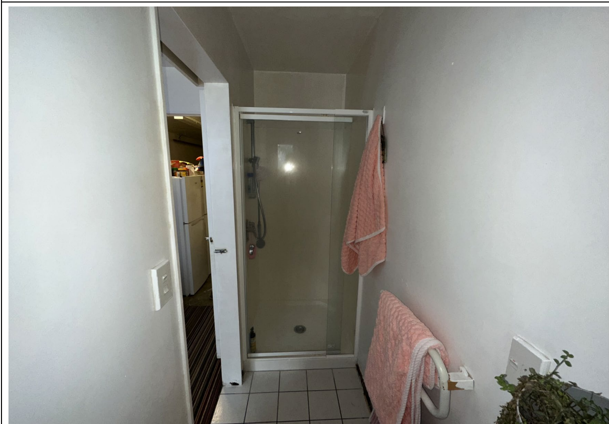
6.18 Overview of Ground Floor Bathroom in Unit 28 facing away from external wall
