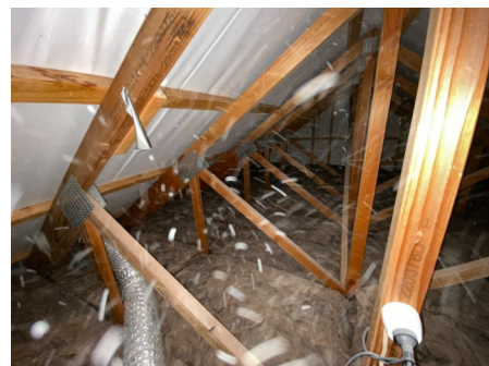
Ceiling Cavity Insulation in good condition and meets the standards. View High Resolution Image Here
