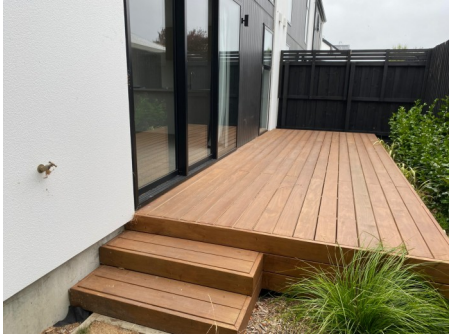
Subfloor surrounds - Rear of property There is no sub floor as the property is built on a concrete foundation. View High Resolution Image Here
