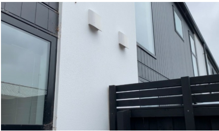
Kitchen extraction system external vent Confirmed by smoke test. View High Resolution Image Here
