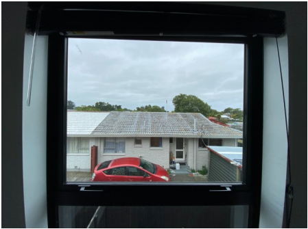
Bedroom 1 The window is compliant for draught stopping. View High Resolution Image Here
