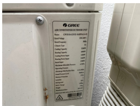
Heater specifications Heater specifications showing an output of 6kW. View High Resolution Image Here
