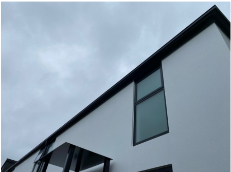
Front of property - spouting Spouting system is in good condition/ or near new condition. View High Resolution Image Here
