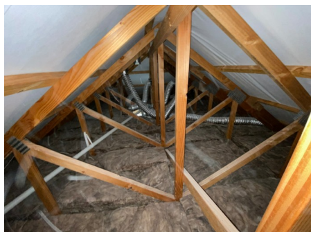
Ceiling Cavity Insulation is evenly distributed throughout ceiling cavity. View High Resolution Image Here
