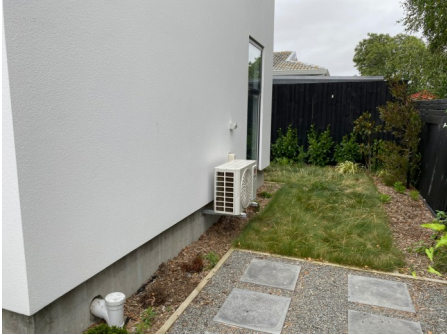
Subfloor surrounds - Right side of property There is no sub floor as the property is built on a concrete foundation. View High Resolution Image Here
