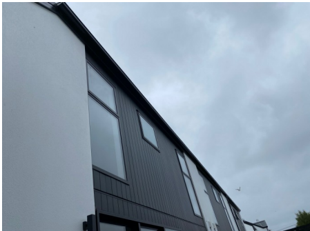
Rear of property - spouting Spouting system is in good condition/ or near new condition. View High Resolution Image Here
