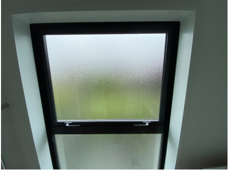
Bathroom 2 The window is compliant for draught stopping. View High Resolution Image Here
