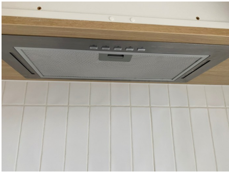
Kitchen extraction system filters The kitchen extraction system filters are free from grease and oil. View High Resolution Image Here
