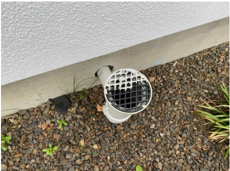
Front of property - soak pit Drain is clear of debris. View High Resolution Image Here
