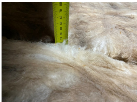
Ceiling Insulation Insulation measurement is 220mm. View High Resolution Image Here
