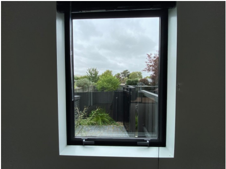
Lounge The window is compliant for draught stopping. View High Resolution Image Here
