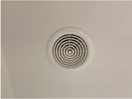
Bathroom 2 extraction system Extraction system vents back into ceiling cavity. View High Resolution Image Here
