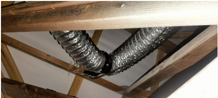
Bathroom 1 Extraction System remediation View High Resolution Image Here 28/02/2025
