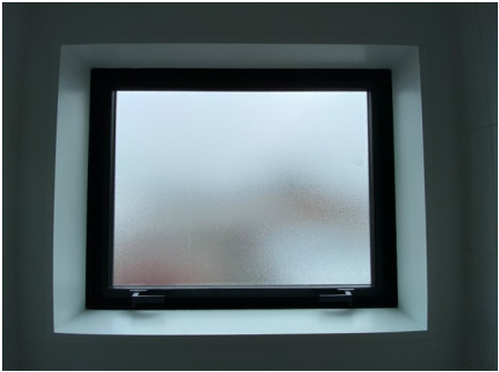
Bathroom 1 The window is compliant for draught stopping. View High Resolution Image Here
