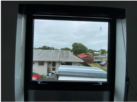
Bedroom 2 The window is compliant for draught stopping. View High Resolution Image Here
