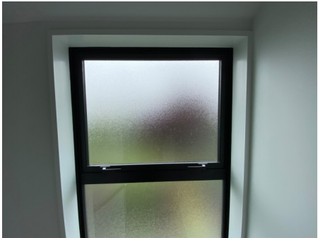
Stairwell The window is compliant for draught stopping. View High Resolution Image Here
