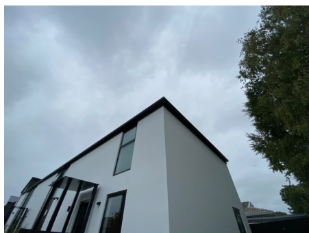
Bathroom 1 extraction system external vent External vent located at the roof. View High Resolution Image Here
