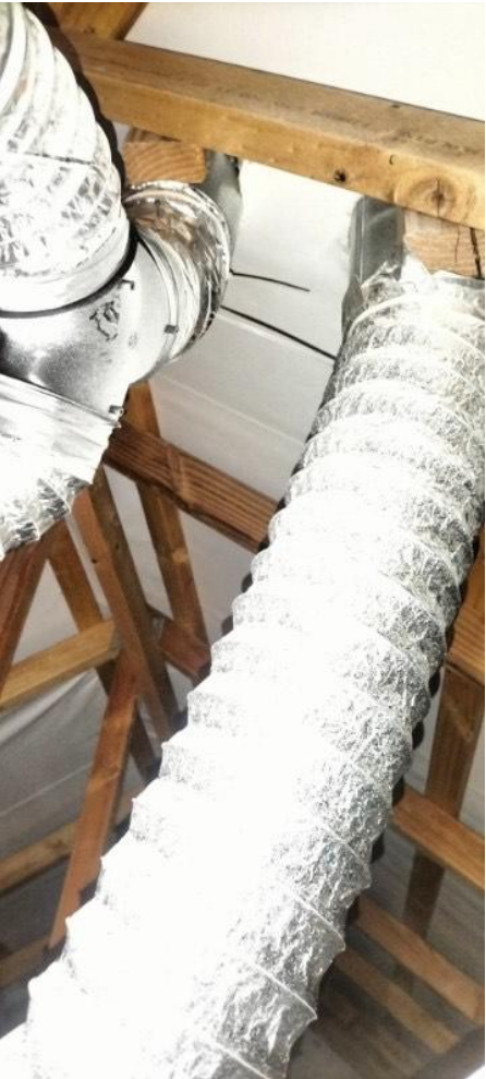
Bathroom 2 Extraction System remediation View High Resolution Image Here 28/02/2025
