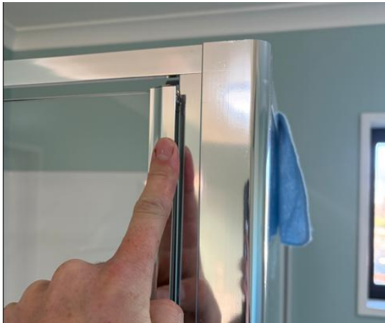
Shower door doesn't easily shut
