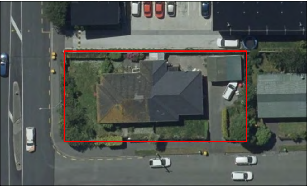
Photo 1G – 2015-2019 aerial imagery shows the chimney has been removed down to roof level.
