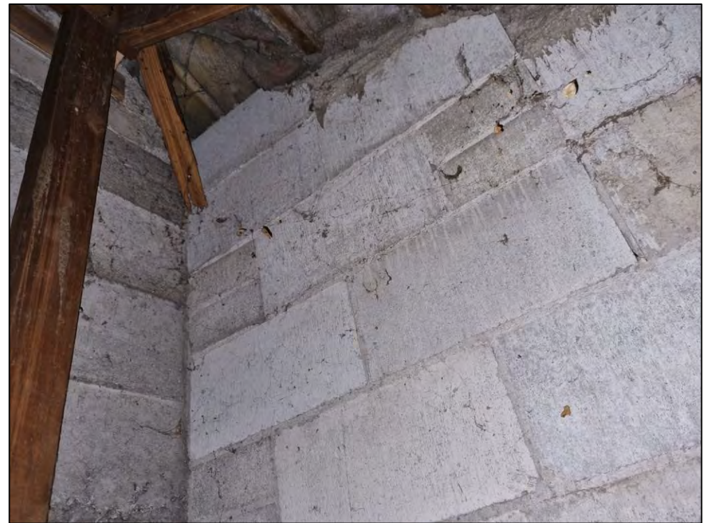
Photo 6D – Newer masonry block wall ( Partition wall extension) above the Laundry extending to the roof tiles constructed circa 1987.
