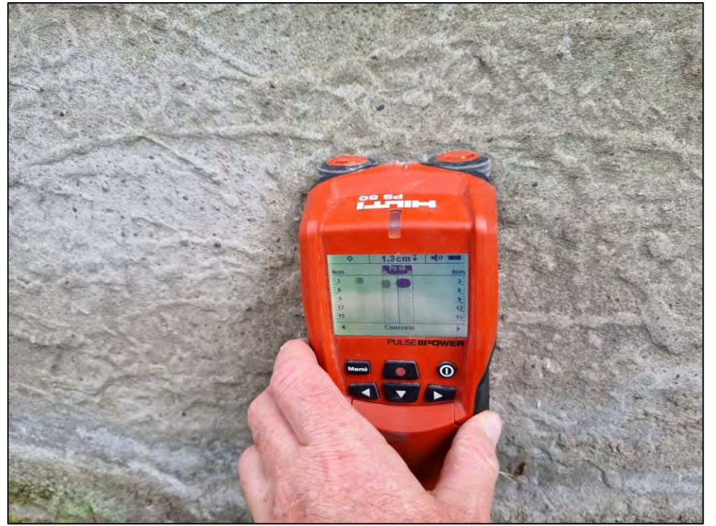
Photo 3D – No reinforcing was detected in the perimeter foundation wall.
