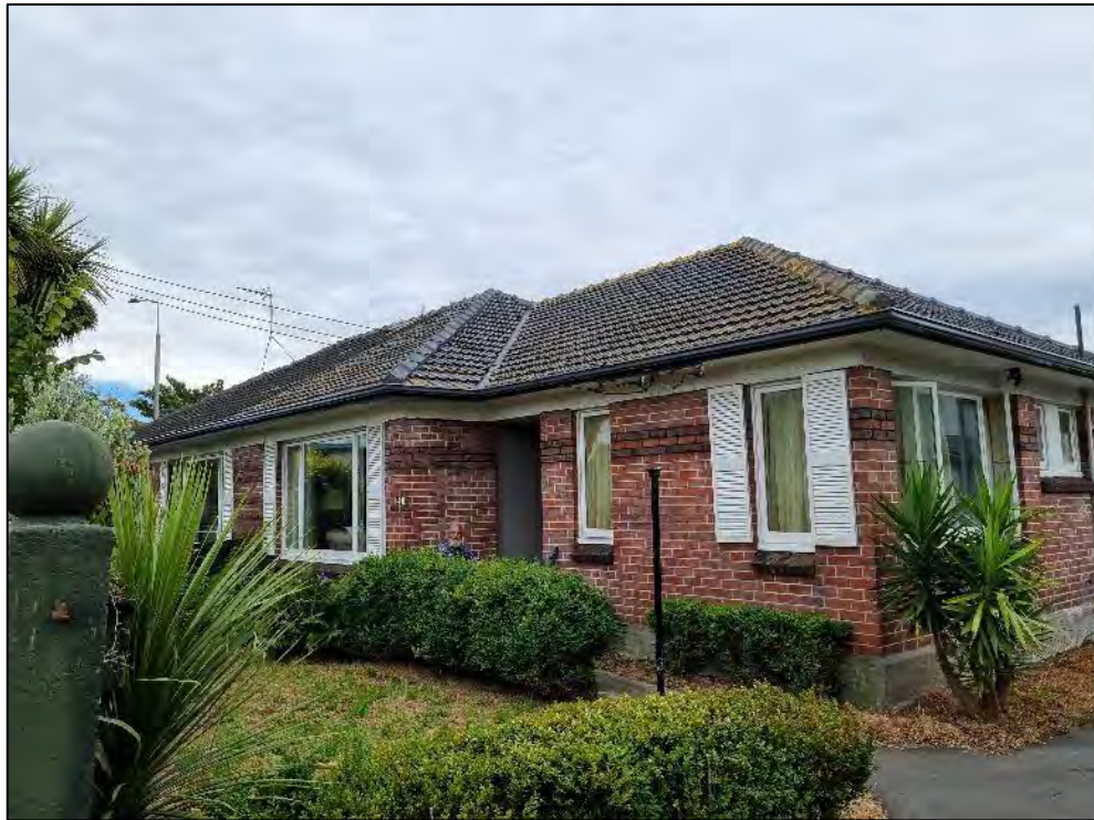
Photo 2A – South elevation (street facing).
