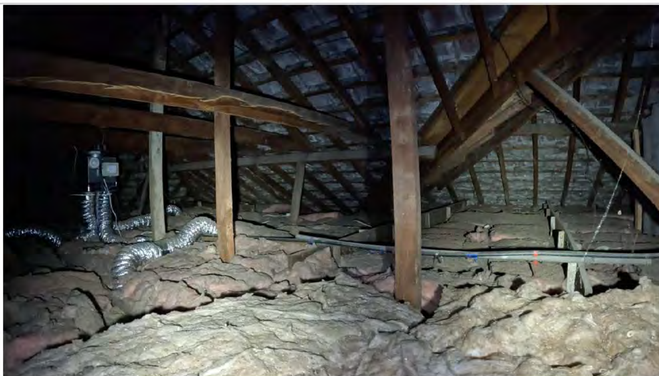
12: The support structure we see in this roof is fairly typical of a roof of this period but does leave some areas vulnerable to sagging.
