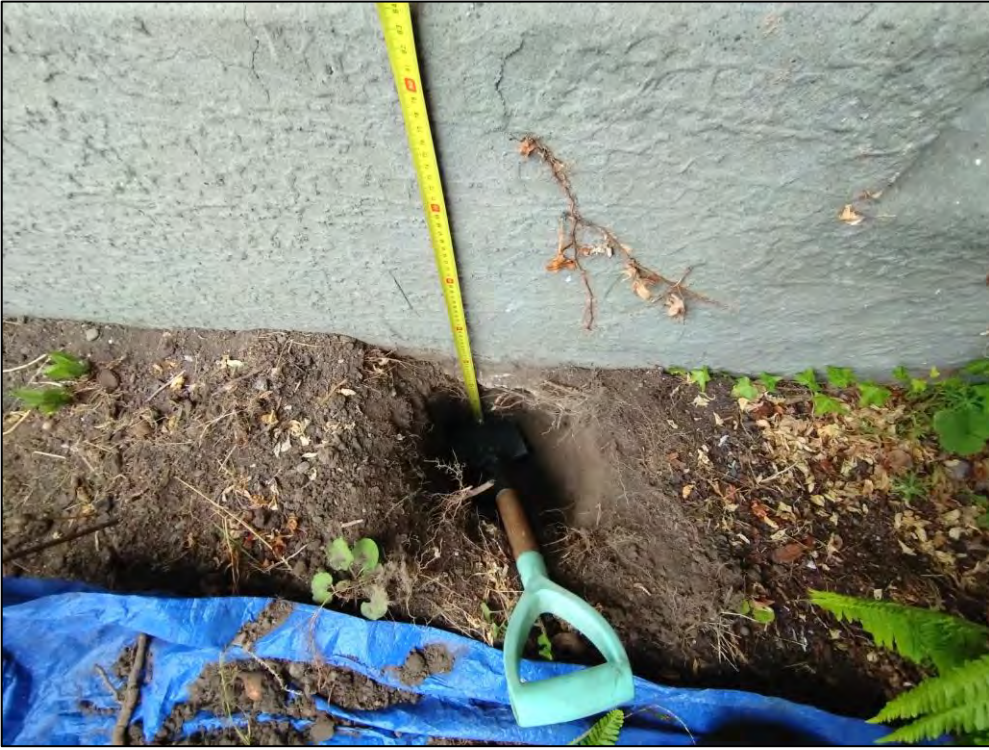
Photo 3A – 350mm Perimeter Foundation embedment depth along the west elevation.
