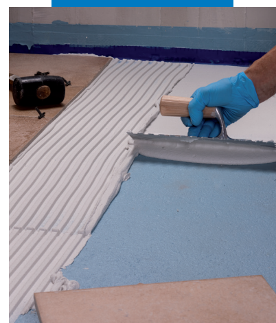
Bonding tiles on Mapelastic AquaDefense
