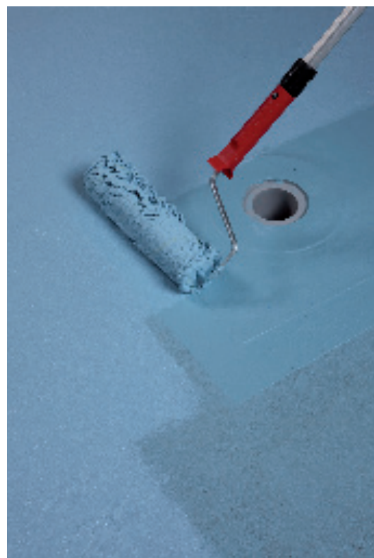
Application of the second coat of Mapelastiq AquaDefense
