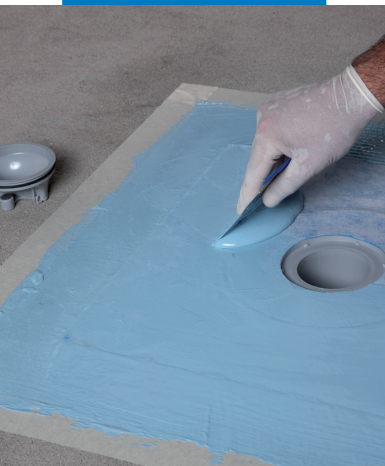
Impregnating Drain Vertical fabric with Mapelastic AquaDefense
