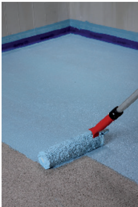
Application of the first coat of Mapelastiq AquaDefense
