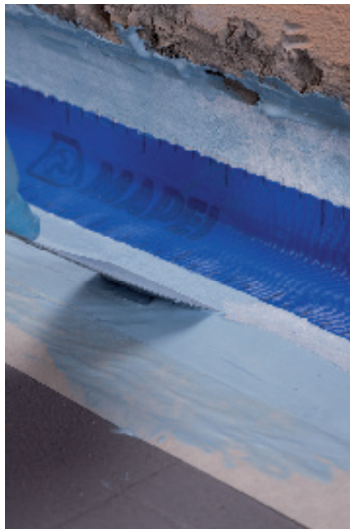
Application of Mapeband to a wall-floor joint with Mapelast AquaDefense
