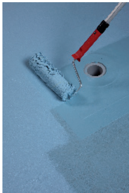
Application of the second coat of Mapelast AquaDefense
