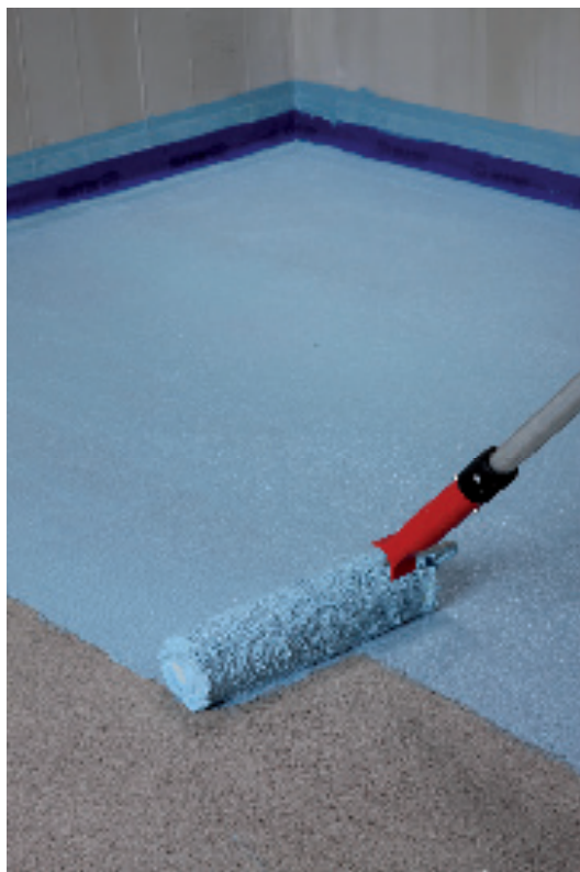
Application of the first coat of Mapelast AquaDefense
