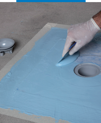
Impregnating Drain Vertical fabric with Mapelastic AquaDefense
