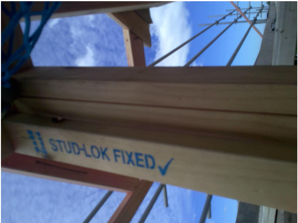
mitek approved framing Taken at 2:09 PM on Monday 19/02/2018
