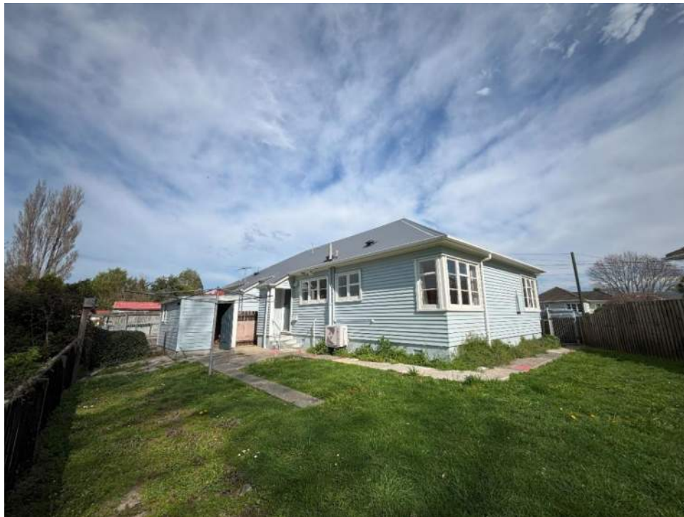
Figure 3: North-east elevation of property, facing the rear corner of 18 Kitchener Place.
