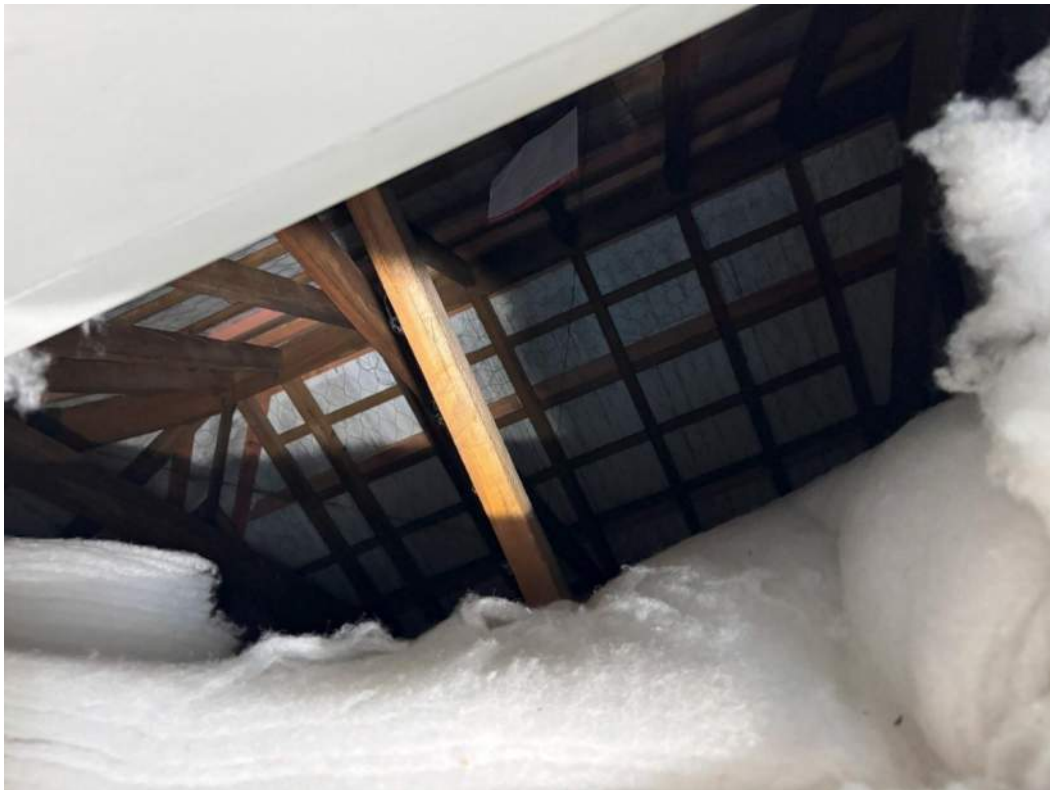
Figure 6: View of the roof structure at 16 Kitchener Place.
