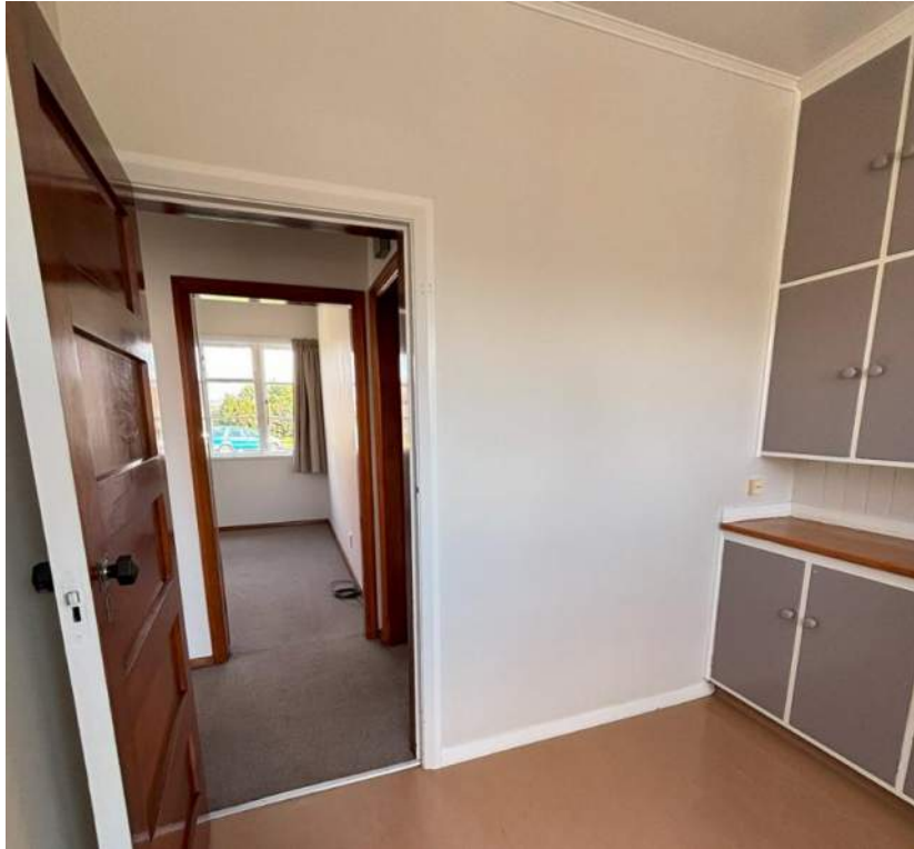
Figure 5: The kitchen-facing side of the internal wall within 16 Kitchener Place to be removed.
