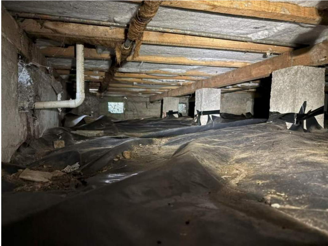
Figure 7: View of the foundation system at 16 Kitchener Place.
