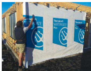
Fix Watergate Plus securely to the frame.
