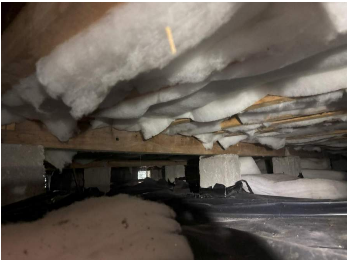
Figure 20: View of the foundation system within 18 Kitchener Place.
