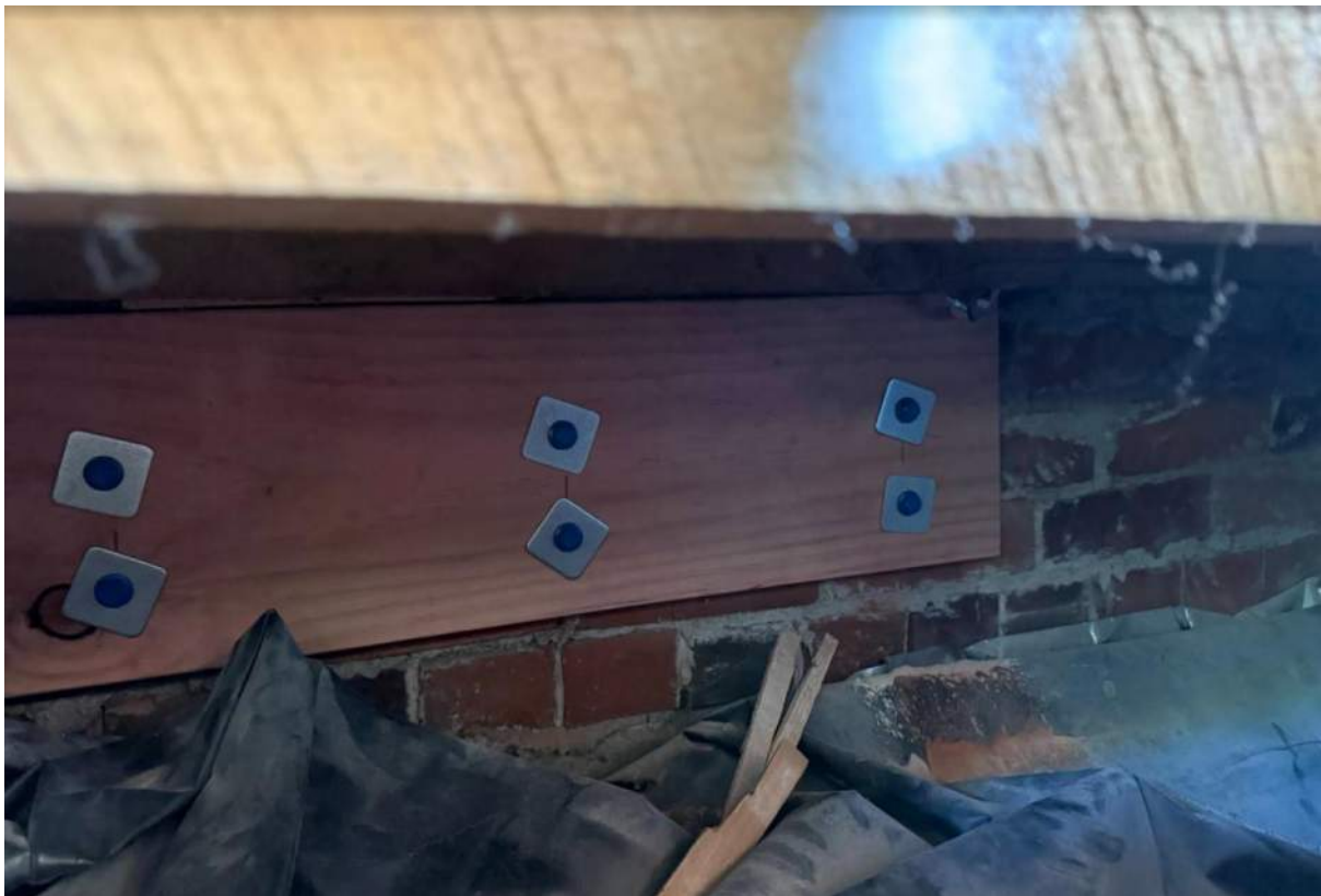
Photo 4: view of ledger support and connection to existing intertenancy wall
