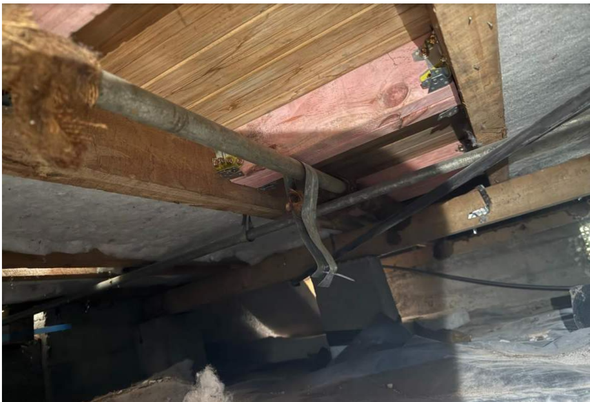
Photo 6: contractor supplied photo of subfloor blocking
