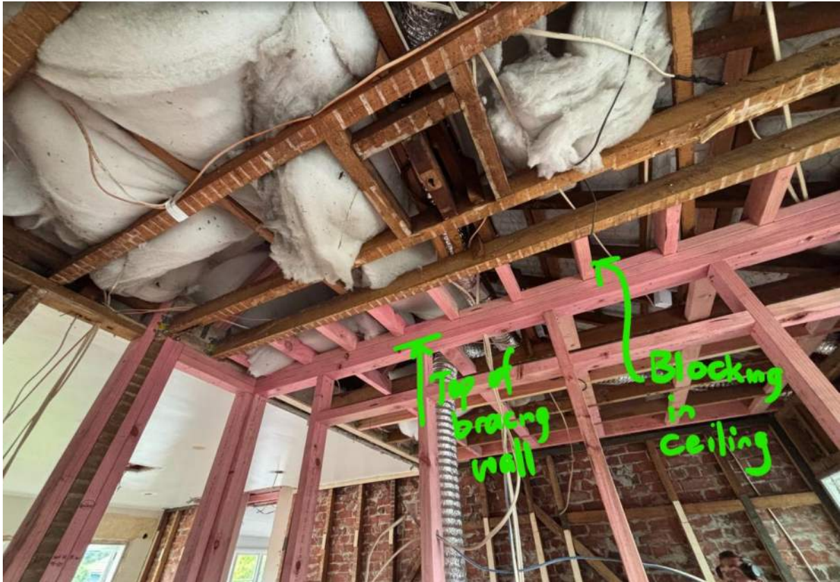
Photo 3: blocking between ceiling joists at top of bracing wall
