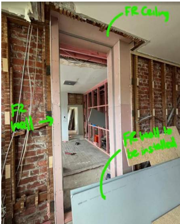
Photo 8: view of chimney infill and FR linings
