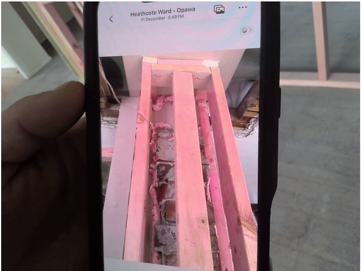
Chimney fill in, GIB Taken at 12:49 PM on Friday 19/12/2025
