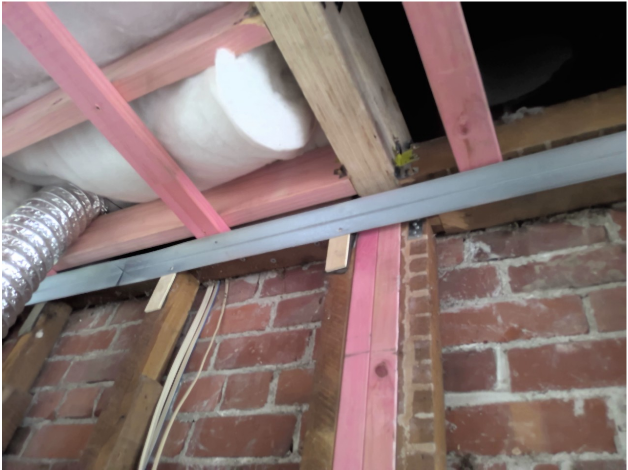
New installed sed LVL Taken at 12:42 PM on Friday 19/12/2025
