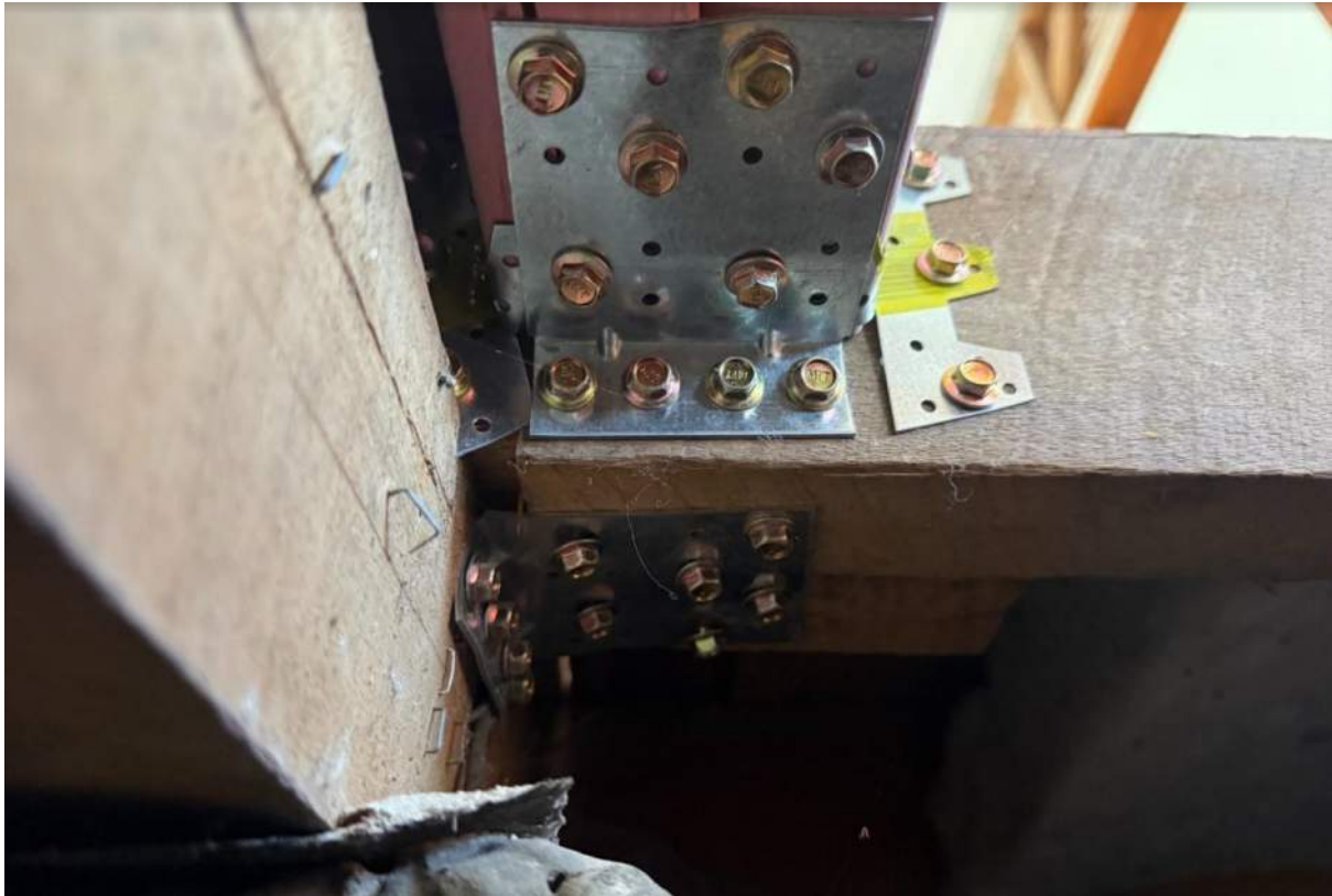
Photo 5: view of connection of blocking in subfloor
