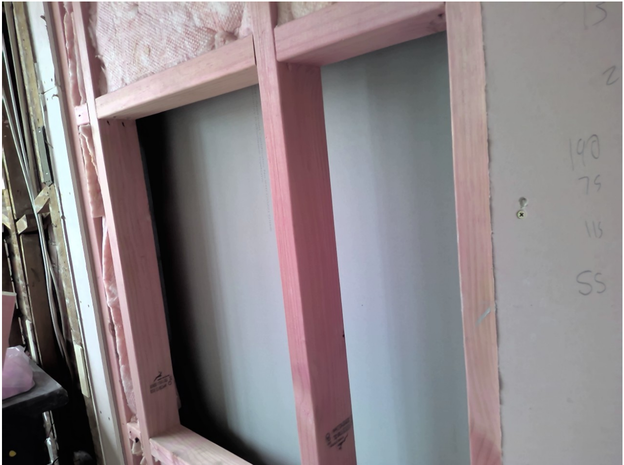
Chimney fill in GIB GBTLAB60 d Taken at 12:51 PM on Friday 19/12/2025
