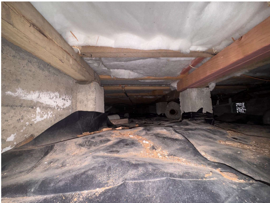
Polyester insulation and polythene ground moisture barrier installed.
