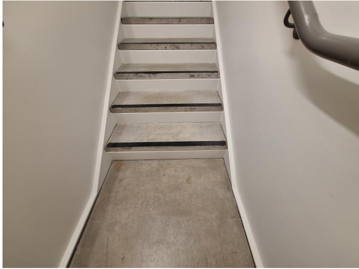
Reset and bed-in loose concrete stair tread – West stair Level 9-10.
