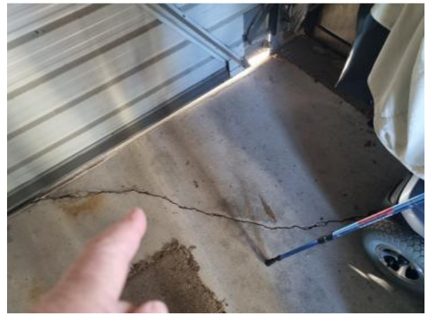
Cracks to garage floor
