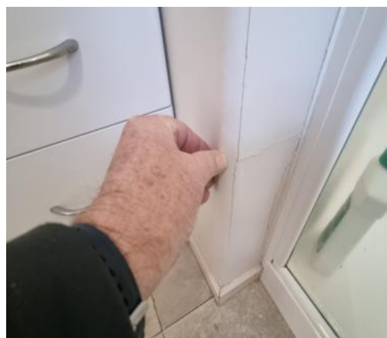
Gib crack bathroom
