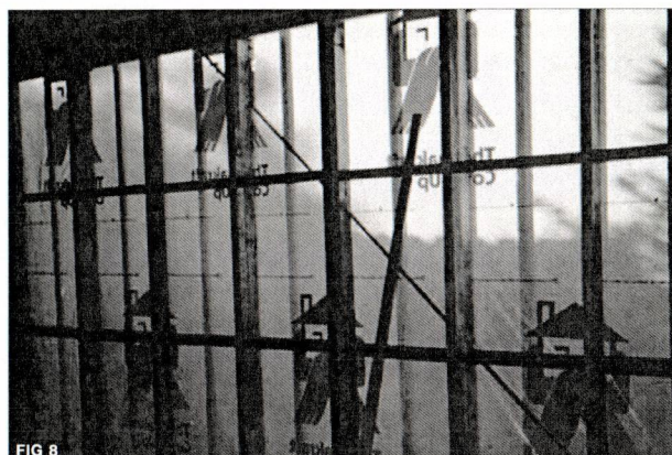
FIG 8 Thermakraft Cover-Up showing the translucent quality and the easy see through, and is resistant to tear in high wind zone till sheathed.
