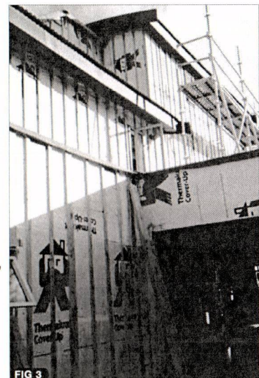
FIG 3 Thermakraft Cover-Up fixed directly to wall framing prior to a 20mm cavity batten is installed.
