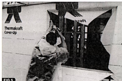
FIG 5 "X" cut Thermakraft Cover-Up and fold back with stapling, preparing for ALUBAND WINDOW SEALING SYSTEM. Simple and efficient.
