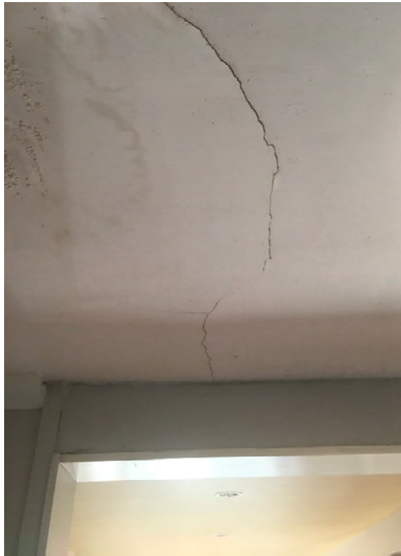
Cracked ceiling lining-previous water damage
