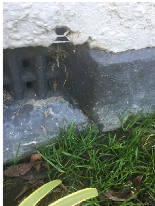
Cracked foundation
