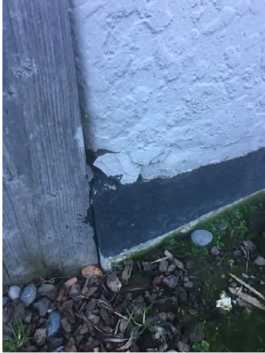
Damaged stucco corner
