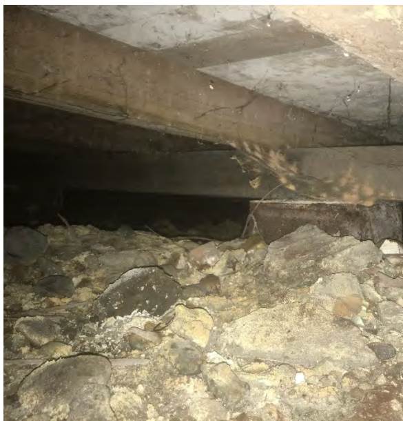
Cracked ceiling lining-previous water damage
