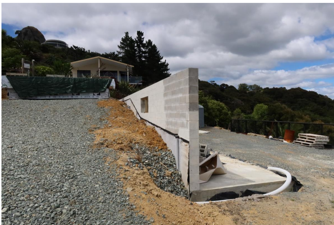
Looking south-west: wall waterproofing an drainage pipe can be seen
