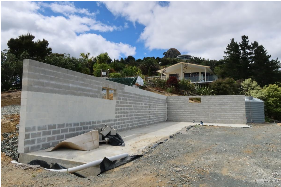
Looking towards south at the existing retaining wall with its footing
