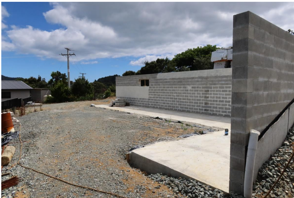
Looking north-east showing existing retaining wall and its footing: wall waterproofing & drainage can be seen
