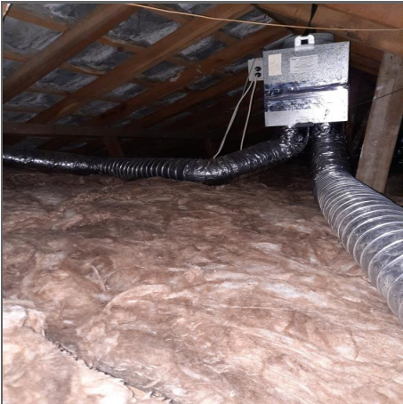
Ceiling - Existing insulation
