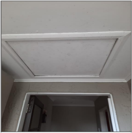
Ceiling - Access to ceiling
