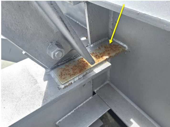
Example of corrosion to steel counterweight structure.
