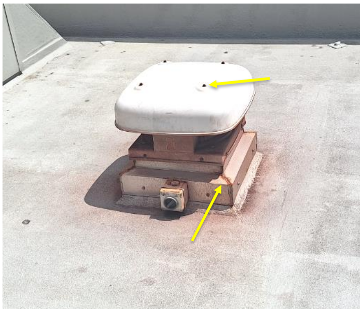
Corroded fixing screws to fan housings. Note early signs of corrosion to flashings.
