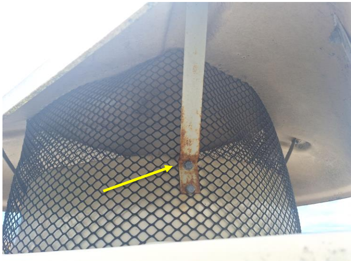
Corrosion to fan housing brackets.
