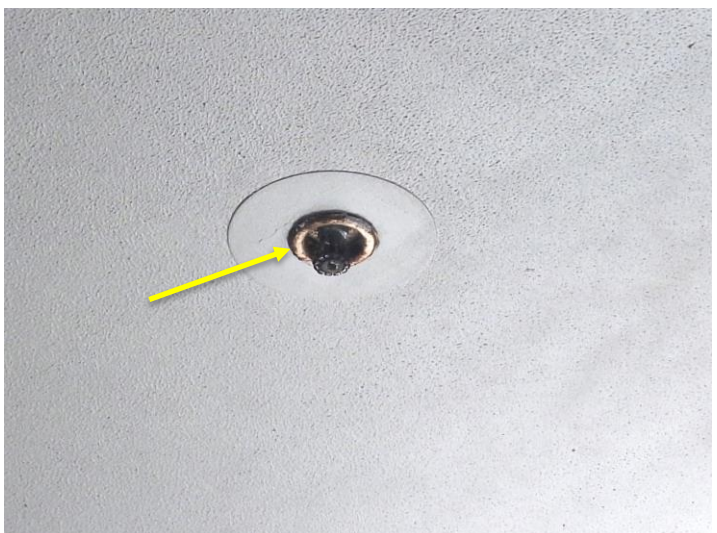
Corroded sprinkler heads to veranda soffit.
