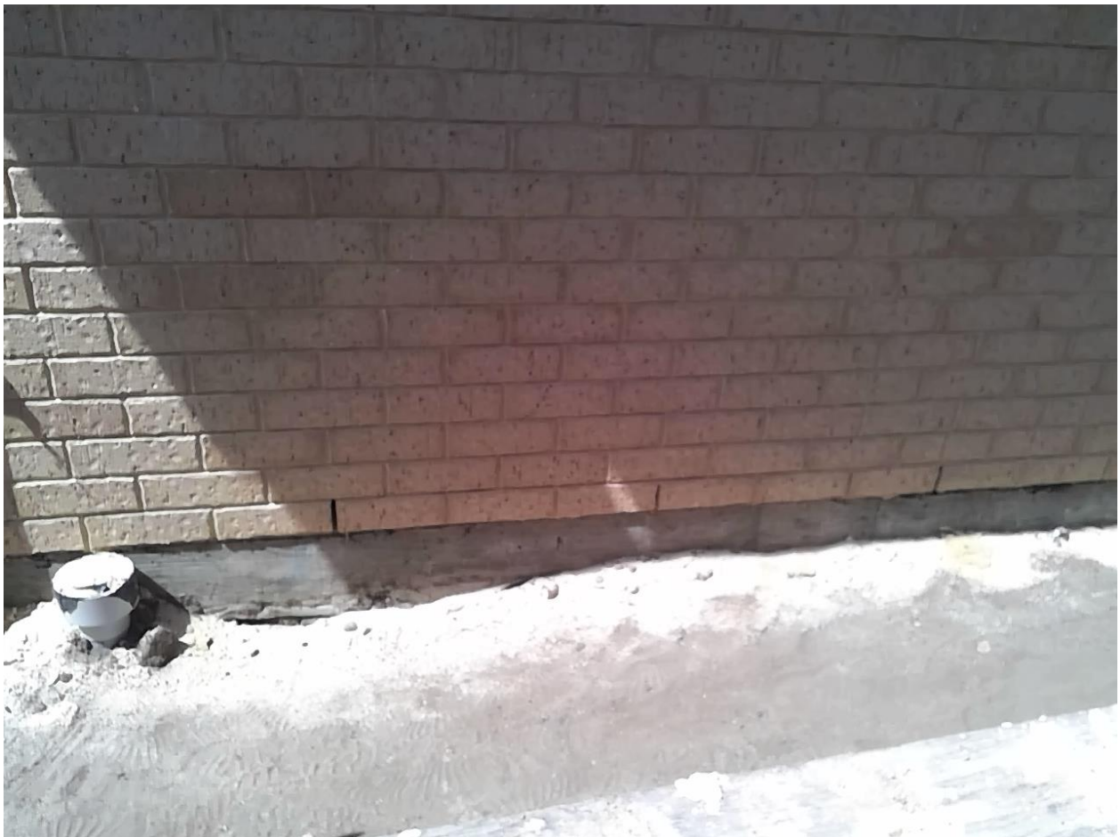
Weep holes every 3rd brick Taken at 12:24 PM on Monday 25/01/2021
