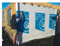
Fix securely to the frame with fasteners such as 6-8mm staples
