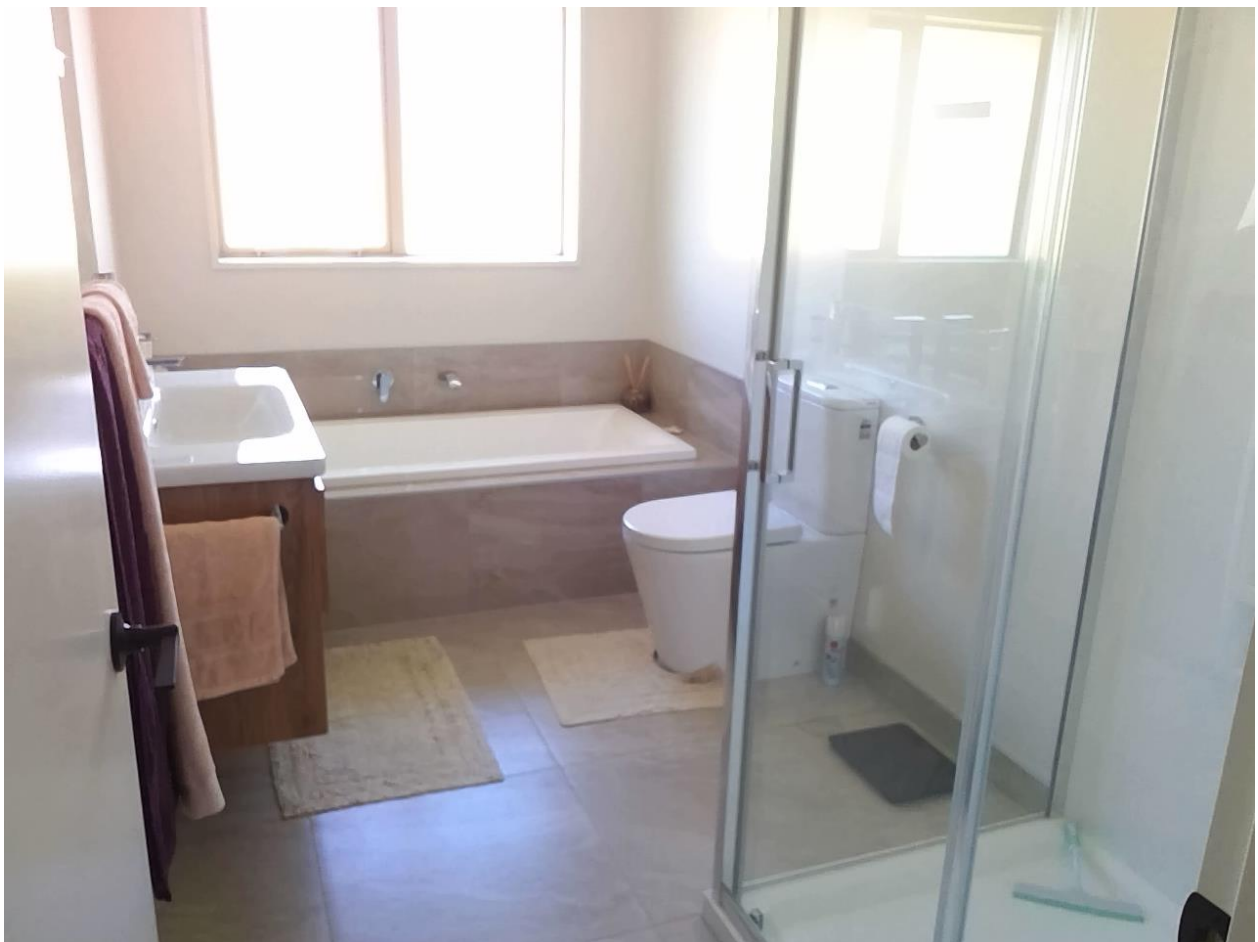
Main bathroom Taken at 1:34 PM on Tuesday 6/04/2021
