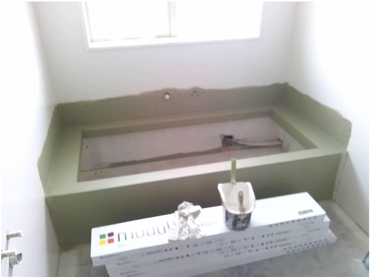
bath cradle waterproofed
