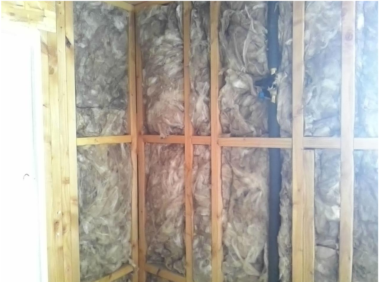
Water isolation valve in garage south wall Taken at 12:28 PM on Tuesday 2/02/2021 Status: Pass
