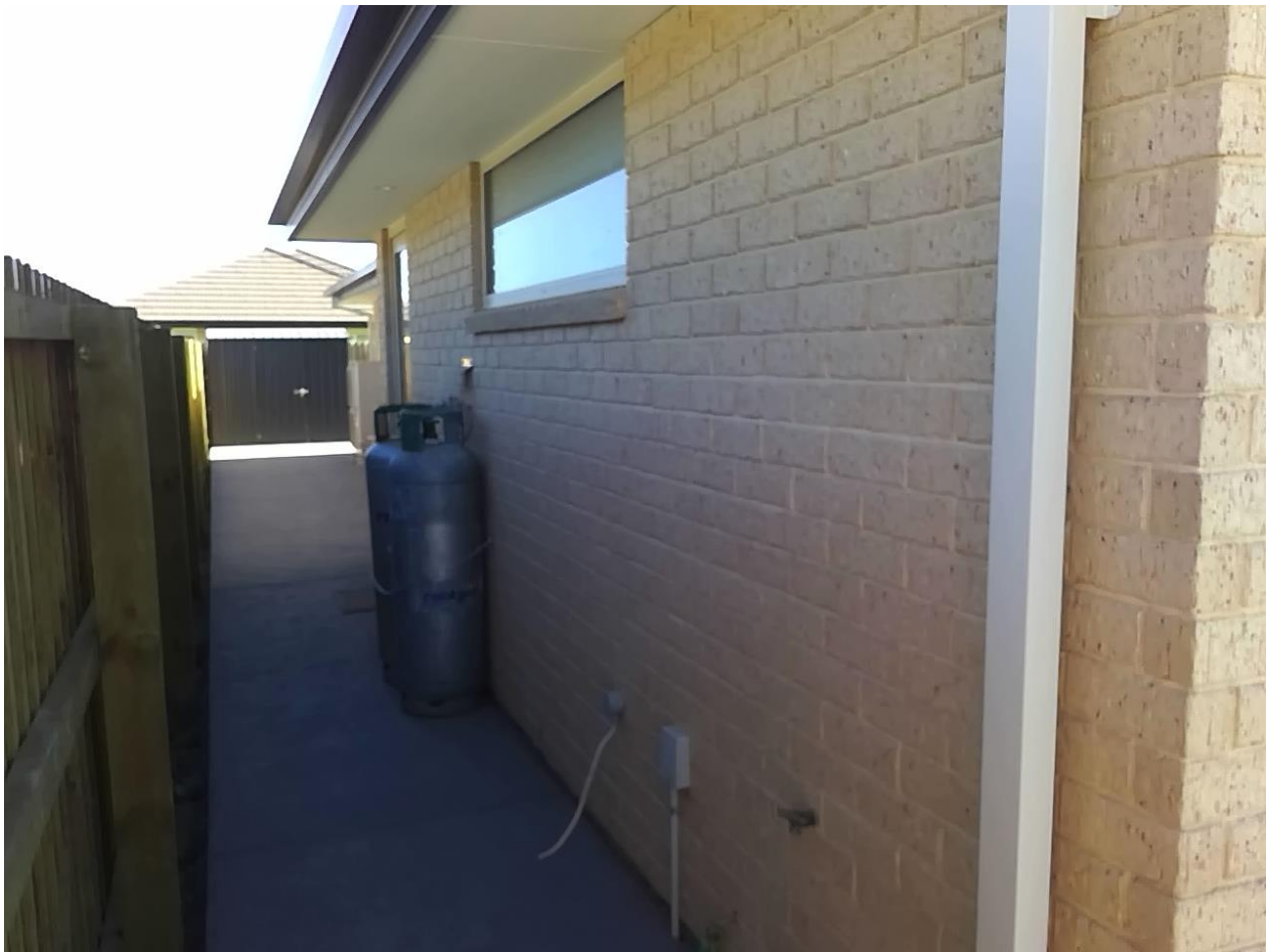
Elevation and gas station Taken at 1:44 PM on Tuesday 6/04/2021
