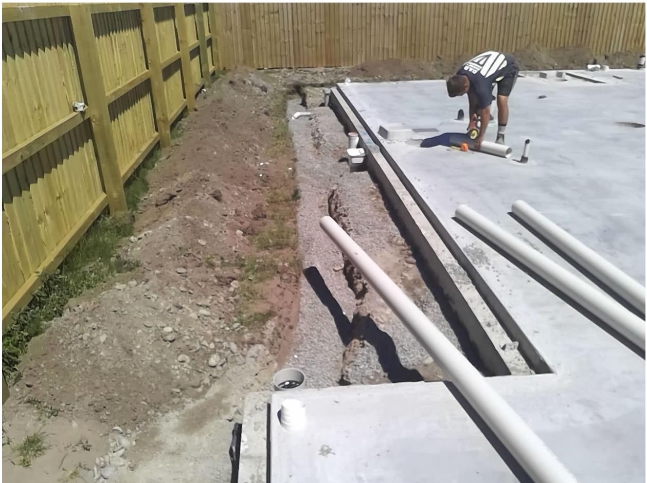
drainage to South ele Taken at 12:00 PM on Monday 16/11/2020 Status: Pass
