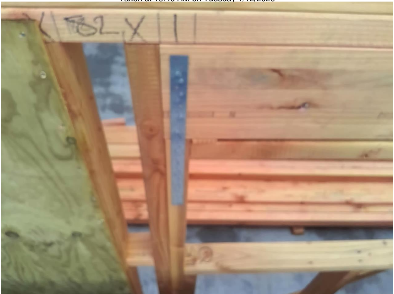
Type G lintel fixings
