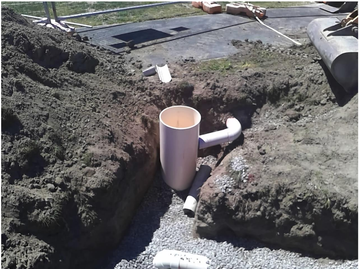
bubbleup connected to kerb Taken at 11:59 AM on Monday 16/11/2020 Status: Pass
