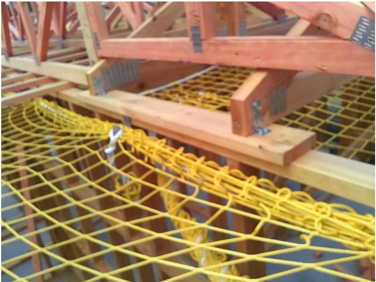
Load bearing wall Taken at 10:47 AM on Tuesday 1/12/2020
