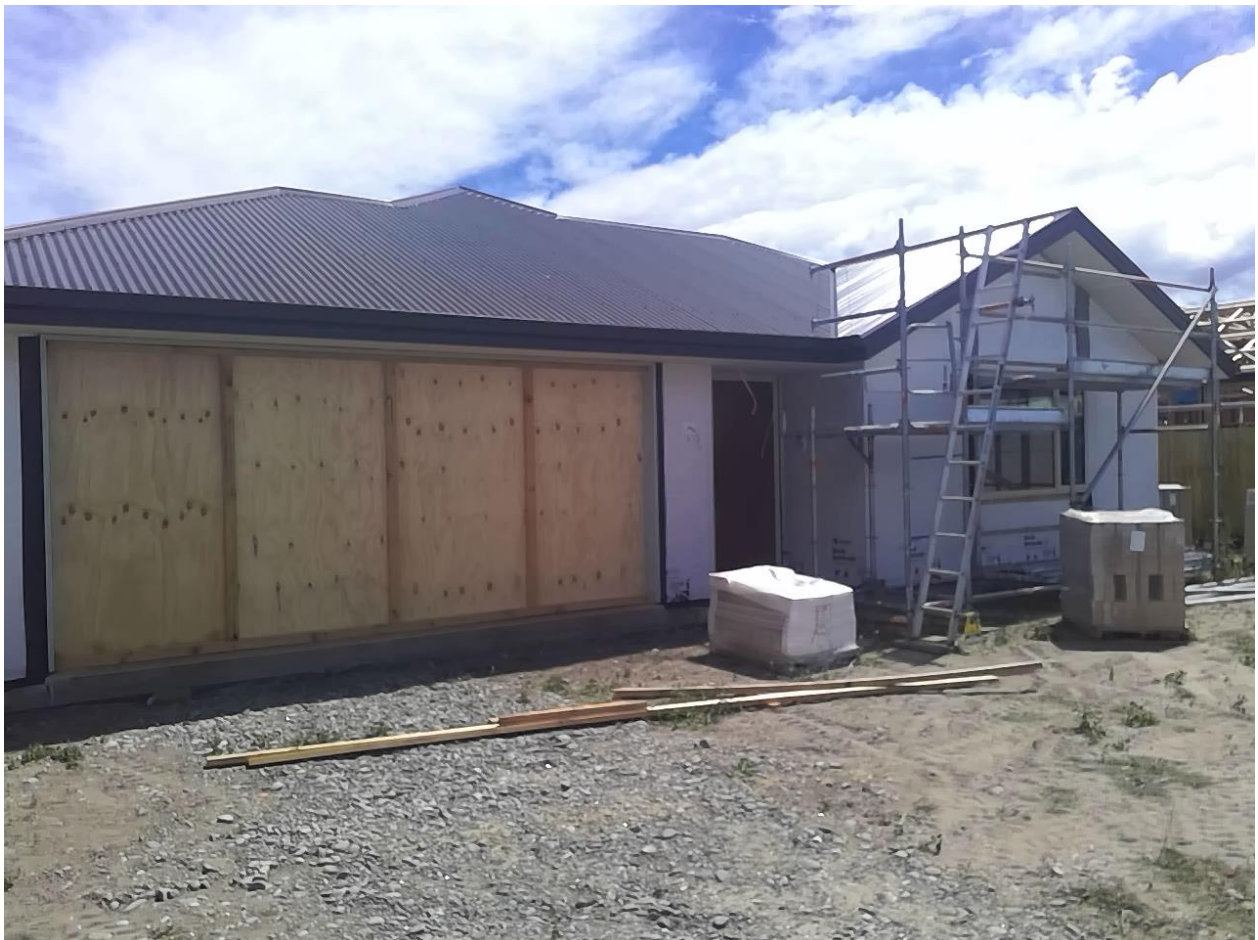
east ele Taken at 2:28 PM on Monday 18/01/2021 Status: Pass
