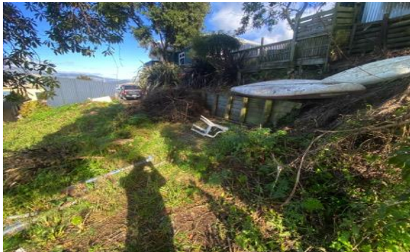
Photo 3: Relatively flat area at the top (west) of the site where there is driveway access. An intact timber post retaining wall is shown on the upslope side.
