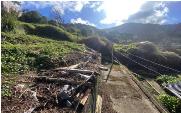
Photo 5: Mass concrete retaining walls on downslope (east) side of the site, appear intact and upright and appear to be owned by the neighbour to the east.
