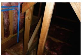
Ceilings are insulated with fibreglass batts, though thickness does not meet Healthy Homes standards. Upgrades may be considered.
