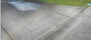
Driveway condition was good, free from major damage, some minor cracking in spots.
